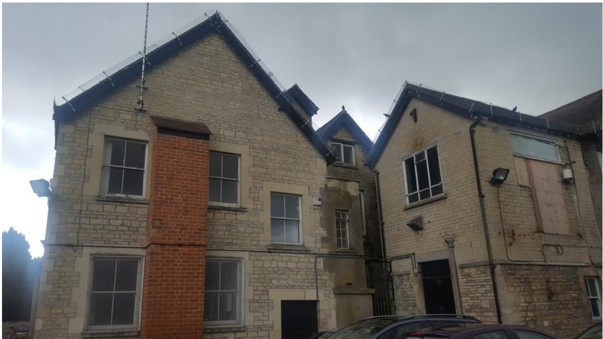
Side (North) Elevations:
