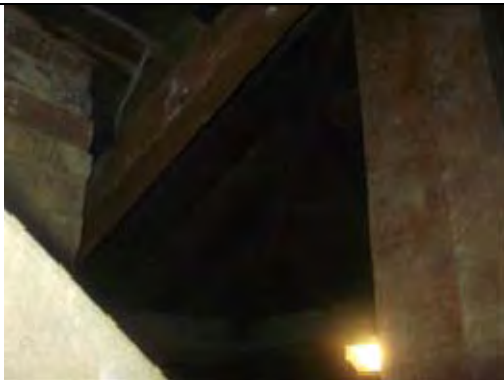
Timber construction to roof
