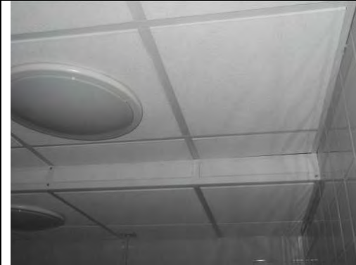
Modern non ACM suspended ceiling tiles
