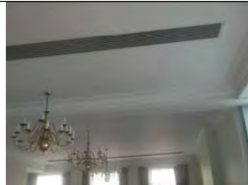
Painted plastered ceiling
