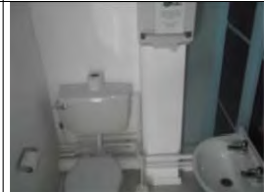
General view of Gents WC
