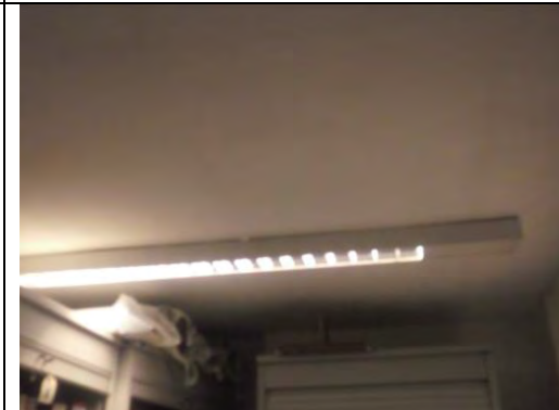
Painted plastered ceiling
