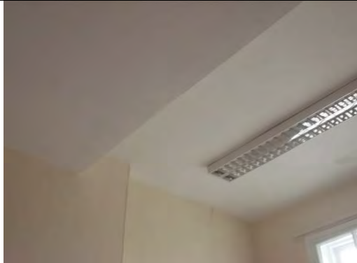
Painted plastered walls and painted plasterboard ceiling
