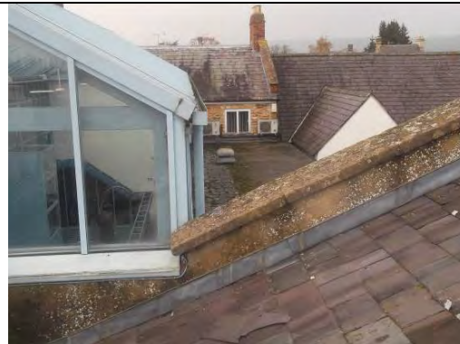
General view of Roof
