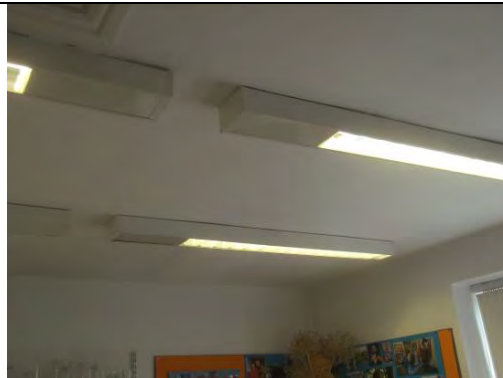
Painted plastered walls and painted plasterboard ceiling
