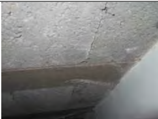
Beam and block construction above
