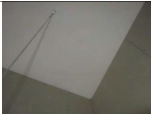
General view above suspended ceiling tiles
