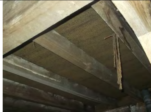
Modern non ACM roofing felt
