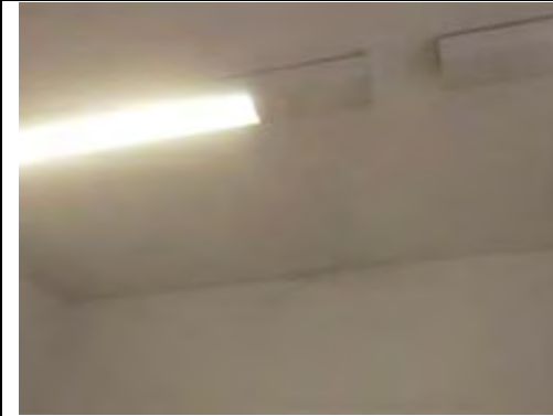
Painted plastered walls and painted plasterboard ceiling
