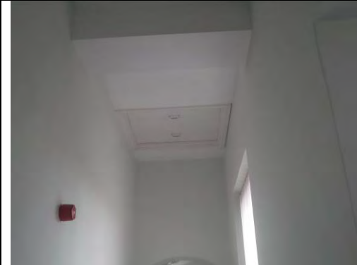
Painted plastered walls
