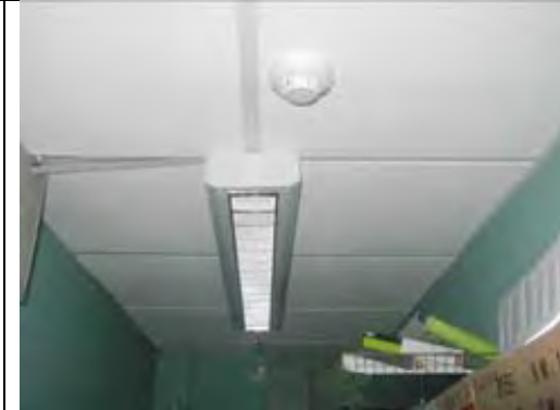
Modern non ACM suspended ceiling tiles
