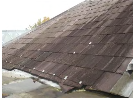
General view of back roof from Skylight
