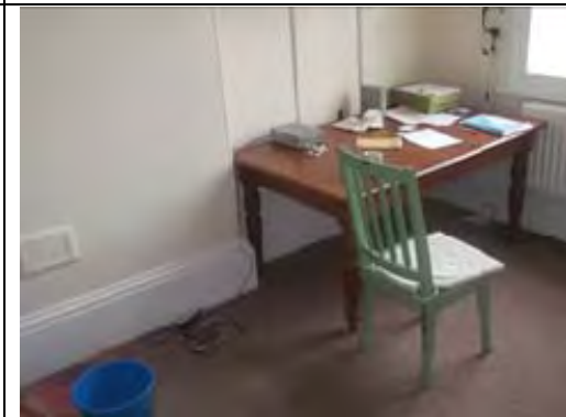
General view of Room 44. Registrar's Office
