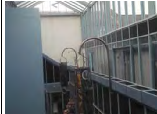
General view of Atrium
