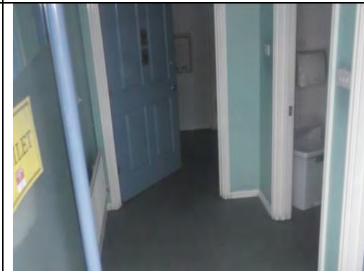
General view of Toilets
