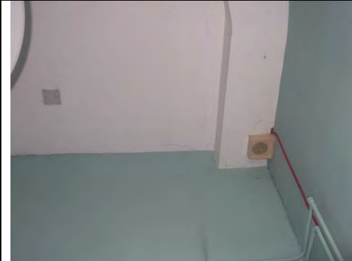
Painted plastered walls and painted plastered ceiling
