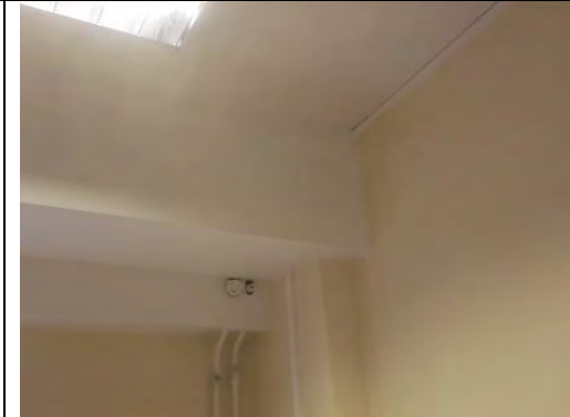
Painted plastered walls and painted plasterboard and timber box work
