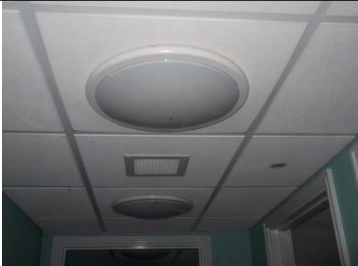
Modern non ACM suspended ceiling tiles
