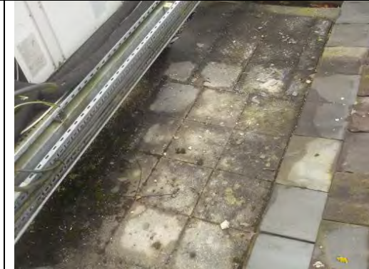
Cement floor tiles and bitumen adhesive to tiles MAOM/5 NADIS
