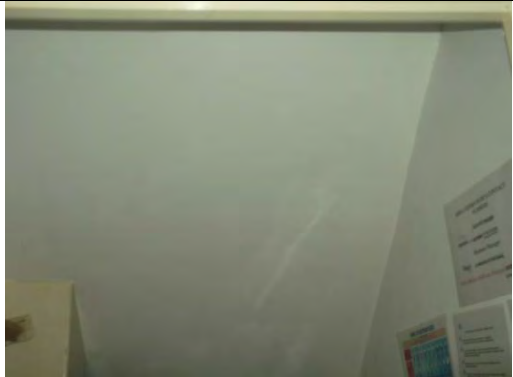
Painted plastered walls and painted plasterboard ceiling
