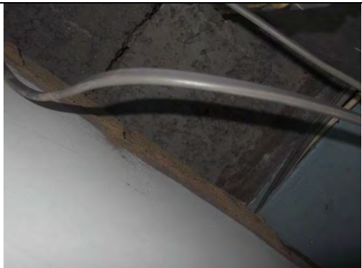
Beam and block floor above suspended ceiling
