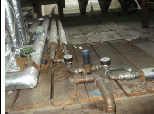
General view within Loft Space
