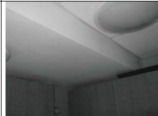
Painted plastered ceiling and modern non ACM suspended ceiling tiles
