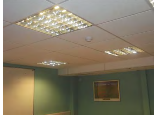
Modern non ACM suspended ceiling tiles
