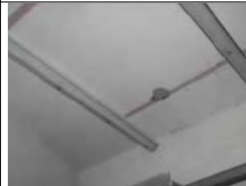
Painted plastered ceiling
