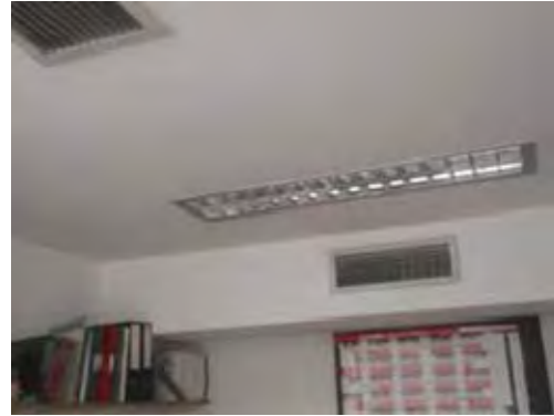
Painted plastered walls and painted plasterboard ceiling
