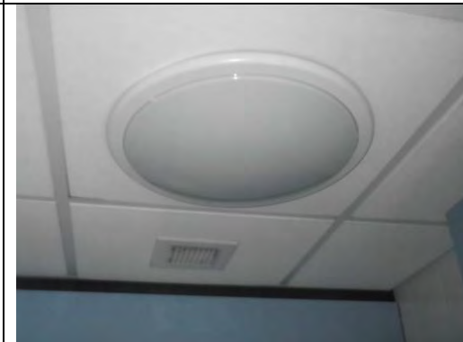
Modern non ACM suspended ceiling tiles
