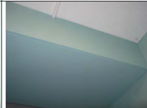
Painted plasterboard and timber box work
