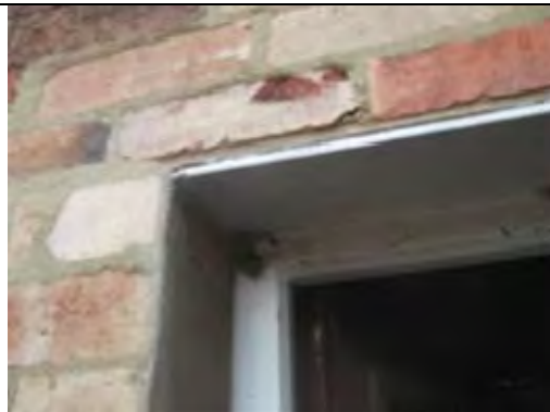
Insulation board above door MAOM/2 NADIS
