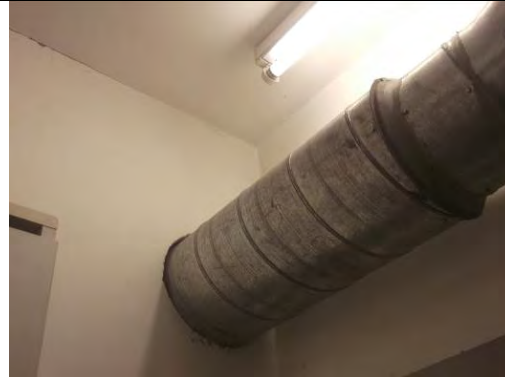
Painted plastered walls and painted plasterboard ceiling
