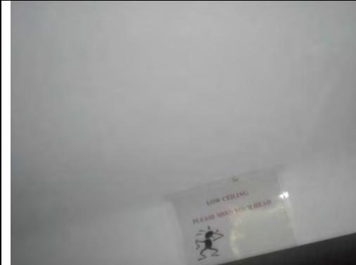
Painted plastered ceiling
