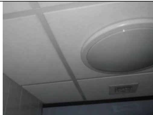
Modern non ACM suspended ceiling tiles
