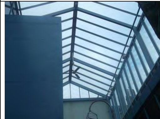
Modern non ACM glass roof lights
