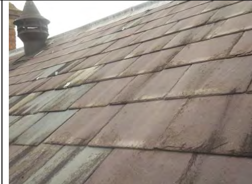
General view of Roof from sky light
