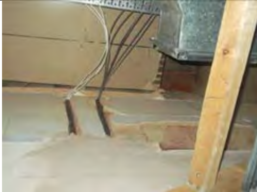
General view above suspended ceiling
