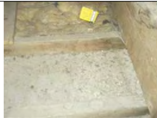
MMMF non ACM insulation to floor
