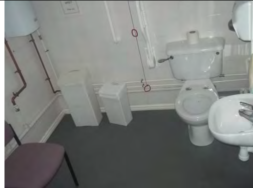
General view of Disabled Toilet
