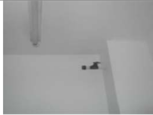
Painted plastered walls and painted plasterboard ceiling
