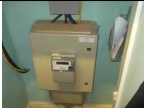
General view within Cupboard
