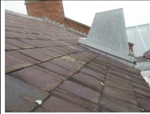
Strongly Presumed cement roof slates intermixed with natural slates Chrysotile
