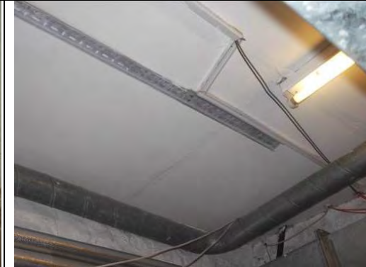
Painted plastered ceiling
