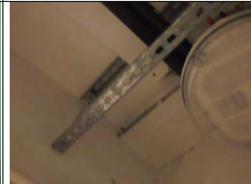
General view above suspended ceiling
