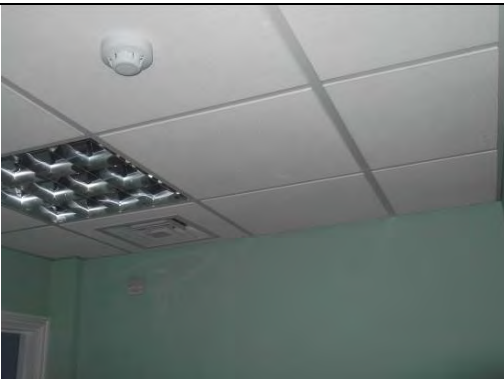
Modern non ACM suspended ceiling tiles
