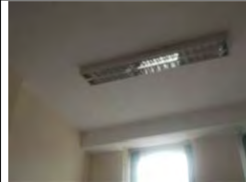
Painted plastered walls and painted plasterboard ceiling
