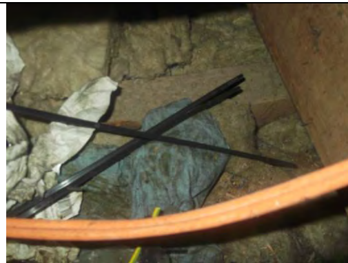
MMMF insulation. Non ACM
