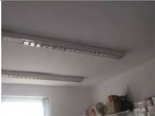
Painted plastered walls and painted plasterboard ceiling
