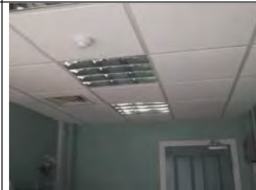
Modern non ACM suspended ceiling tiles
