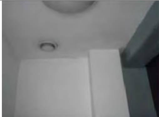
Painted plastered walls and painted plasterboard ceiling. Non ACM boxwork
