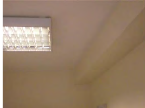
Painted plasterboard and timber box work
