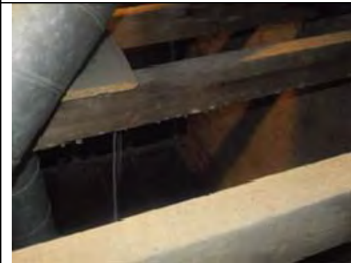
Timber construction to roof
