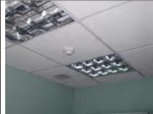
Modern non ACM suspended ceiling tiles
