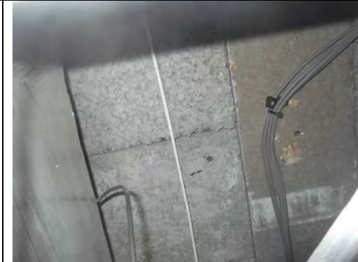
Beam and block above suspended ceiling tiles
