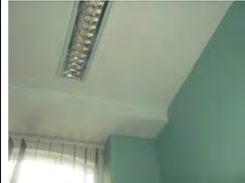
Dry lined internal walls and painted plastered ceiling
