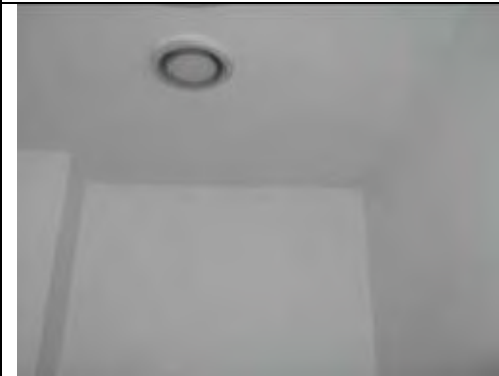
Painted plastered walls and painted plasterboard ceiling
