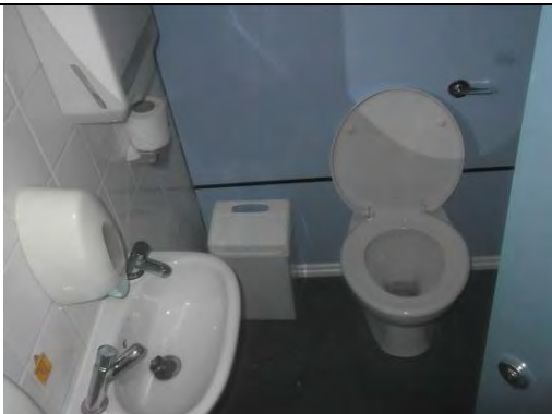
General view of Ladies Toilets
