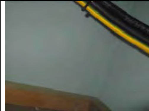
Painted plastered walls
