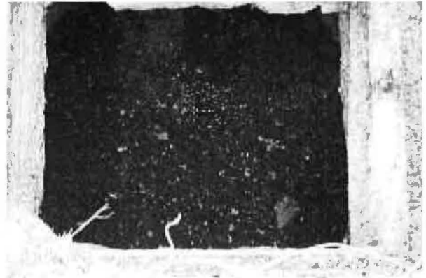
D-20 Dug-well at Manor Farm: interior backfilled
