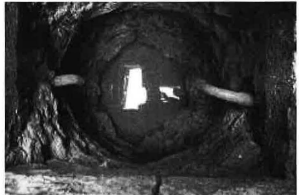
D-22 Dug-well at Riverdale: interior
