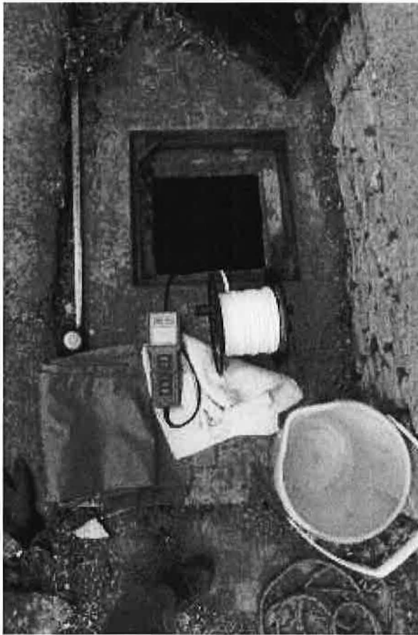
D-15 Well-head at Coln House West
