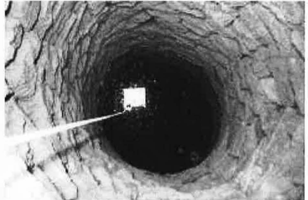
D-14 Well interior at Coln House West
