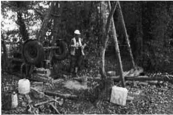
D-9 Drilling Borehole B5
