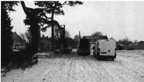
D-7 Drilling Borehole A2
