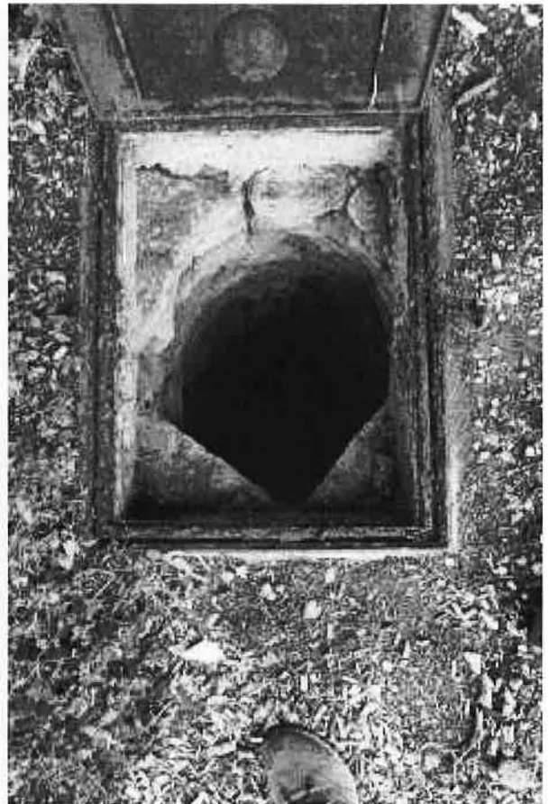
D-16 Well-head at 2 Dynevor Place
