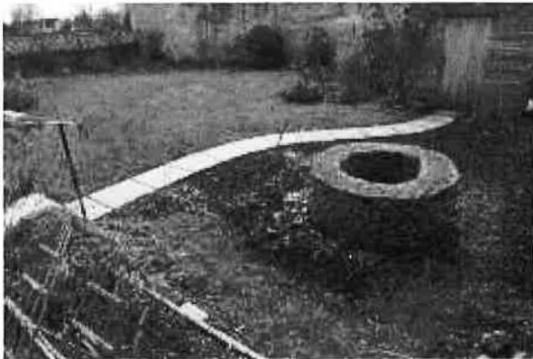
D-19 Dug-well at Comrie: well-head
