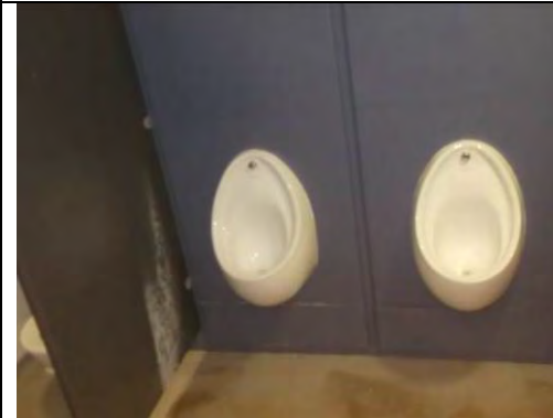
General view of Gents WC
