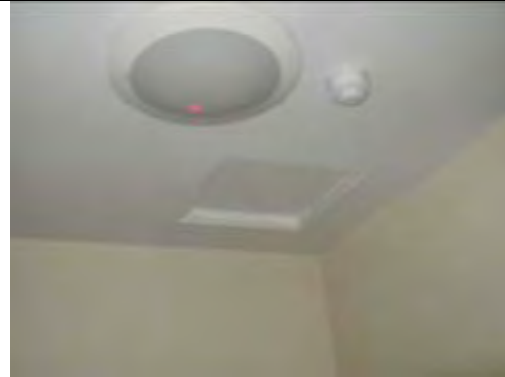
Painted plastered walls and painted plasterboard ceiling
