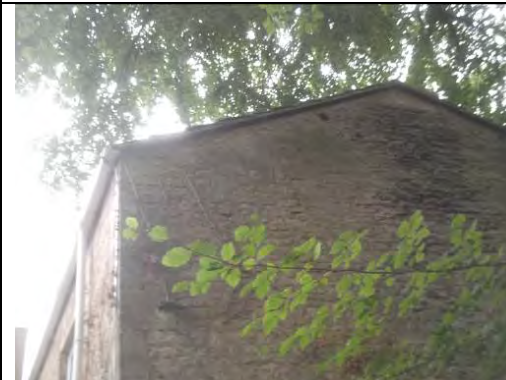
Cement under clocking to roof VS to CDCOTR/1 Chrysotile
