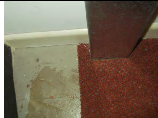
Carpet on concrete
