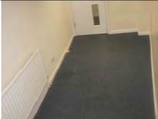
General view of Corridor
