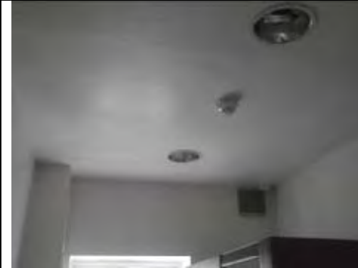
Painted plasterboard ceiling and painted plastered walls
