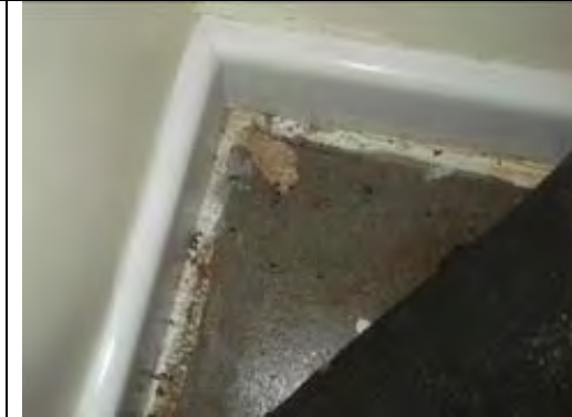
Carpet on concrete
