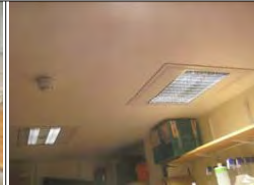
Painted plasterboard ceiling
