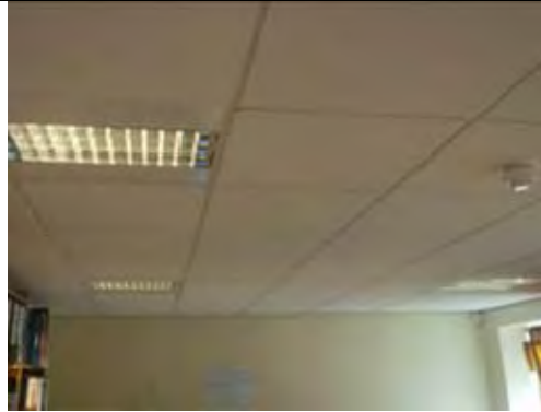
Modern non ACM suspended ceiling tiles and painted plastered walls
