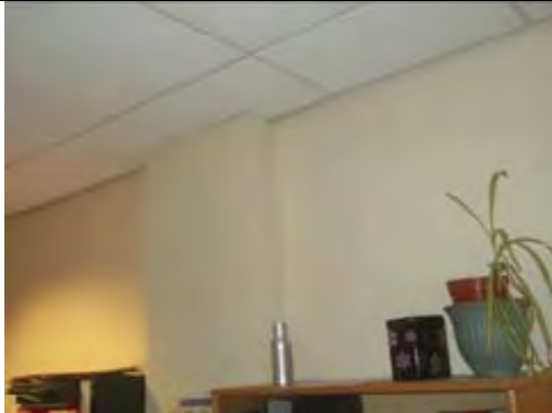
Painted plastered walls
