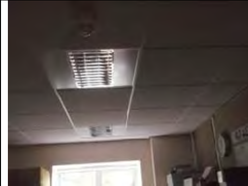
Modern non ACM ceiling tiles
