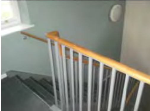
General view of Stairwell
