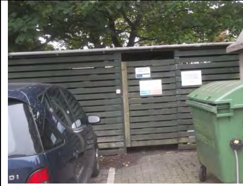
Timber walls to Bike Shed
