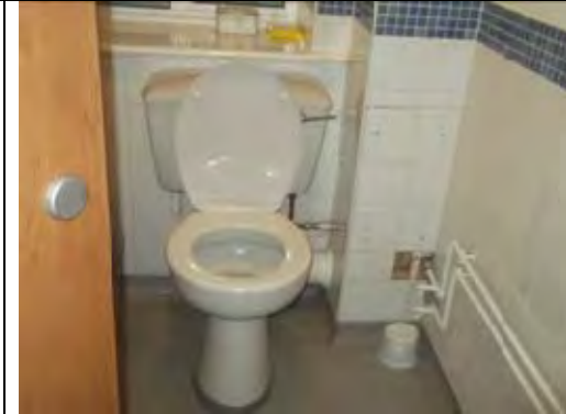
General view of Ladies Toilet
