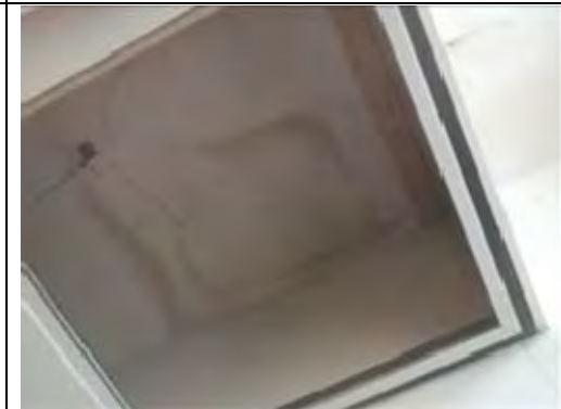
Painted plastered ceiling
