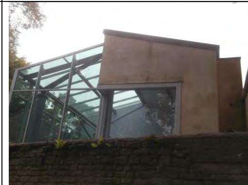
Rendered wall and non ACM end capping sheet
