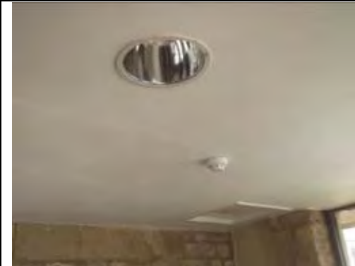
Painted plasterboard ceiling and stone walls
