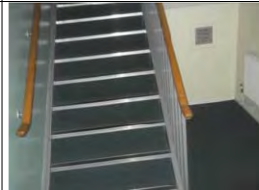
General view of Stairwell
