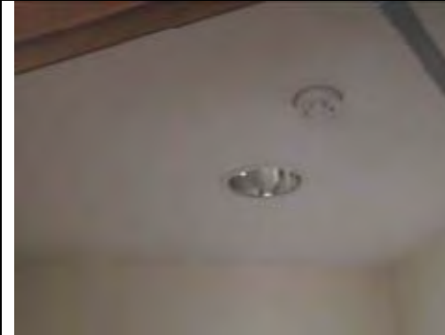
Painted plasterboard ceiling and solid painted walls and painted plasterboard walls
