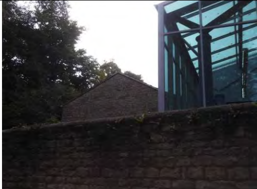
Cement under cladding to roof VS to CDCOTR/1 Chrysotile
