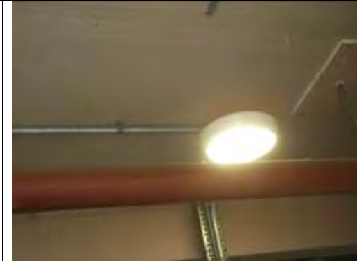
Painted plastered ceiling
