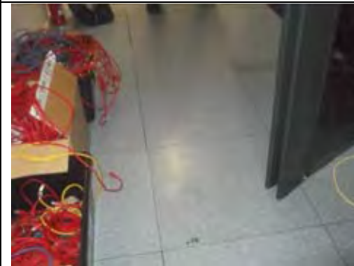
Modern non ACM timber suspended floor with non ACM antistatic flooring
