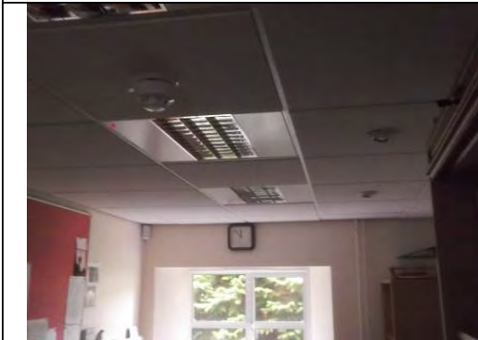
Modern non ACM suspended ceiling tiles and painted plastered walls
