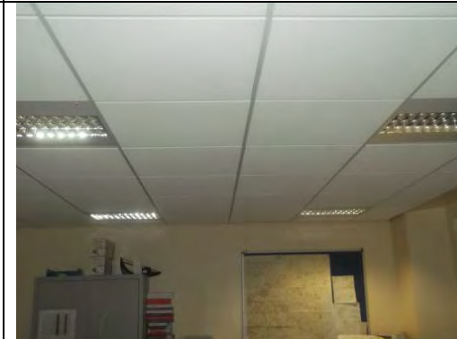
Modern non ACM suspended ceiling tiles
