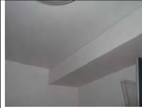
Painted plastered ceiling
