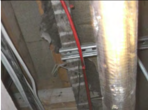
General view above suspended ceiling
