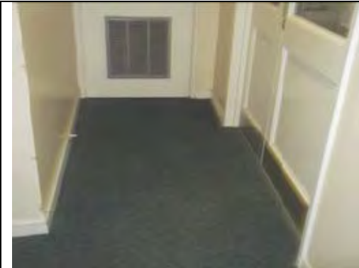
General view of Corridor
