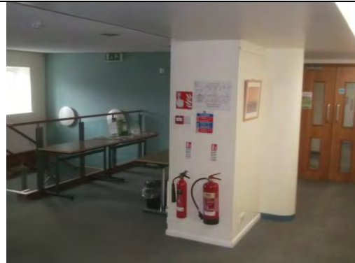
General view of area outside Council Chambers
