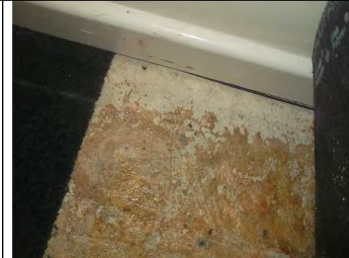
Concrete floor below carpet tiles
