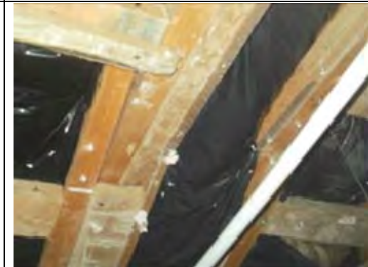
General view above suspended ceiling
