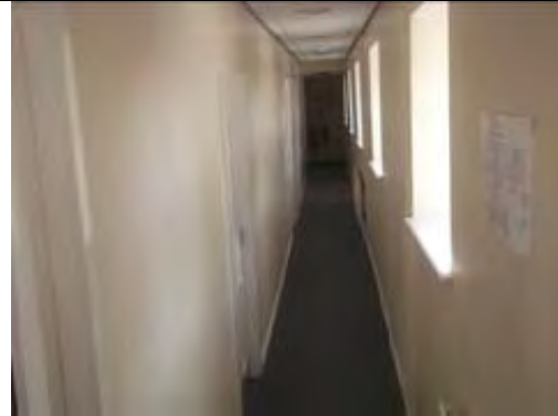
General view of Corridor
