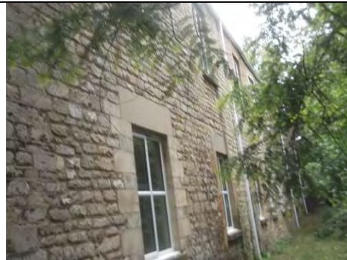
Stone walls and plastic rainwater goods
