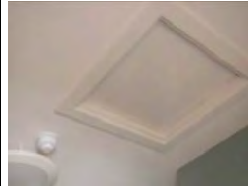
Painted plasterboard ceiling
