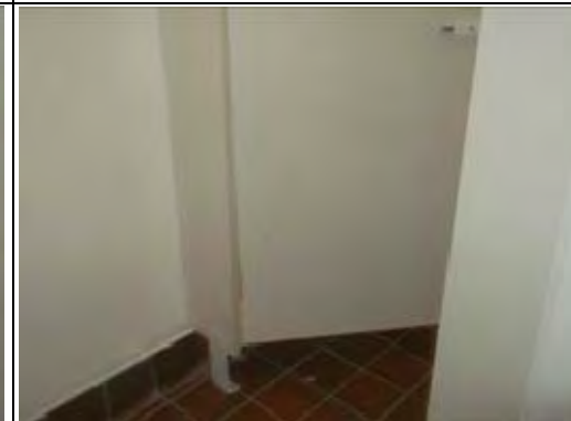
General view of Ladies Toilets
