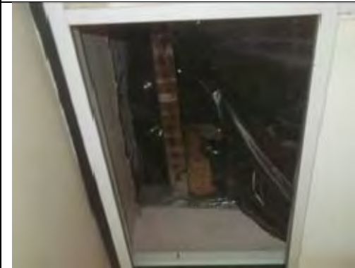
General view above suspended ceiling
