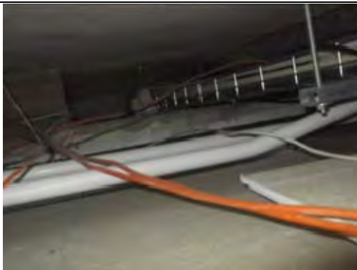
General view above suspended ceiling tiles
