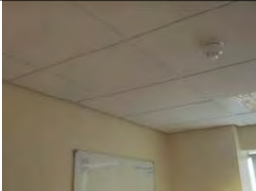
Modern non ACM suspended ceiling
