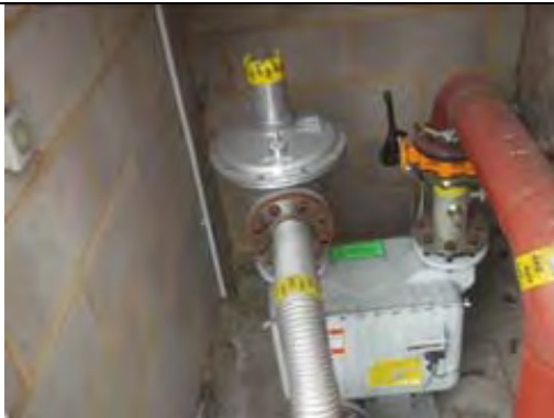
General view of Gas Meter House
