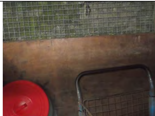
Timber lining to walls
