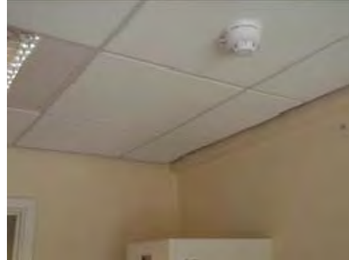
Modern non ACM suspended ceiling tiles
