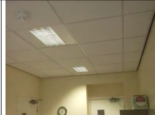
Modern non ACM suspended ceiling tiles
