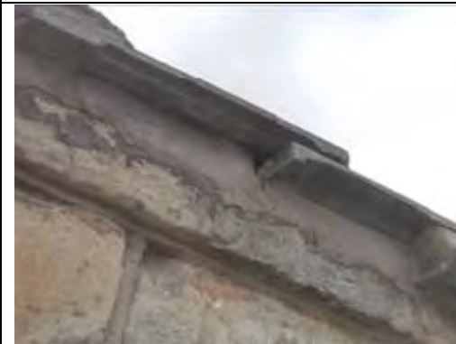
Concrete roof tiles
