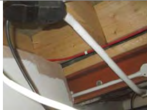
General view above suspended ceiling tiles
