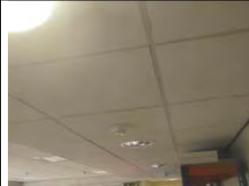
Modern non ACM suspended ceiling tiles
