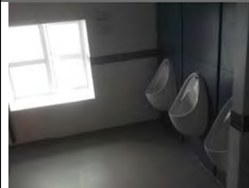
General view of Gents Toilet
