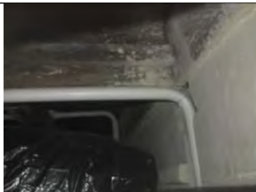
MMM insulation within plastic wrap above suspended ceiling tiles
