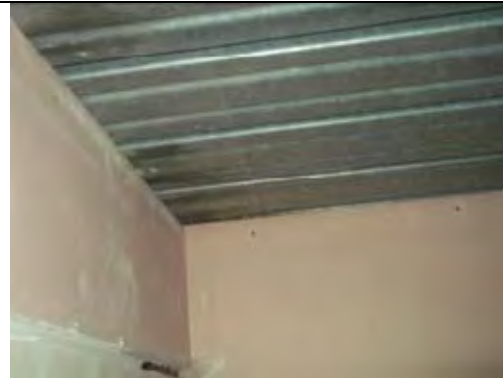
Metal profiled sheet to ceiling above suspended ceiling
