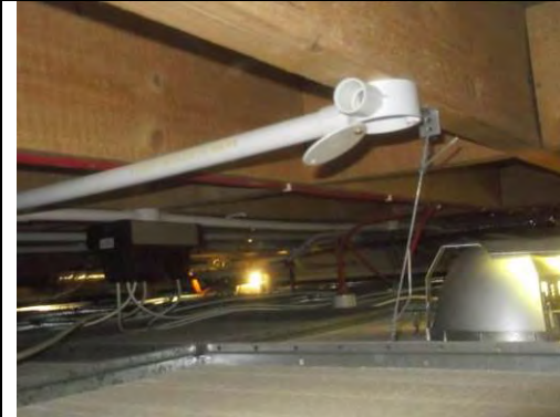
General view above suspended ceiling
