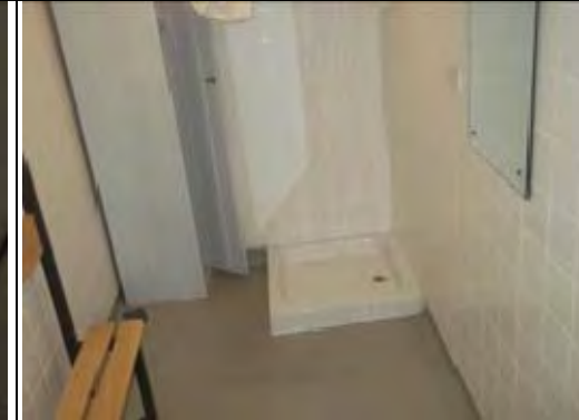
General view of Shower Room. Modern non ACM shower
