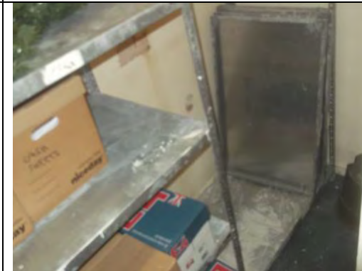
Painted plastered walls
