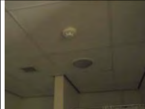
Modern non ACM suspended ceiling tiles
