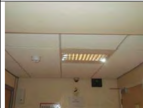
Modern non ACM suspended ceiling tiles and painted plastered walls
