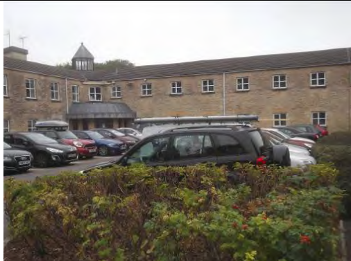
General view of Offices
