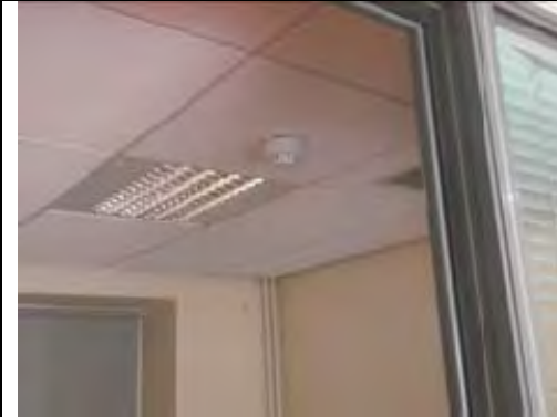
Modern non ACM suspended ceiling tiles
