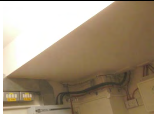
Painted plasterboard to ceiling
