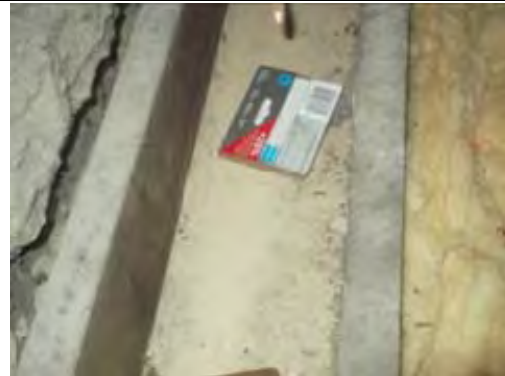
MMMFI insulation above plasterboard ceiling
