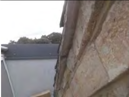
Cement under cloaking to roof CDCOTR/1 Chrysotile
