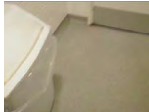
Modern non ACM flooring
