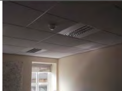
Modern non ACM suspended ceiling tiles and painted plastered walls and painted plasterboard walls
