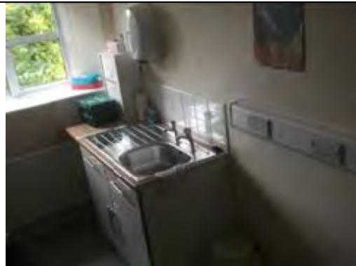
General view of First Aid Room. Modern non ACM kitchen unit
