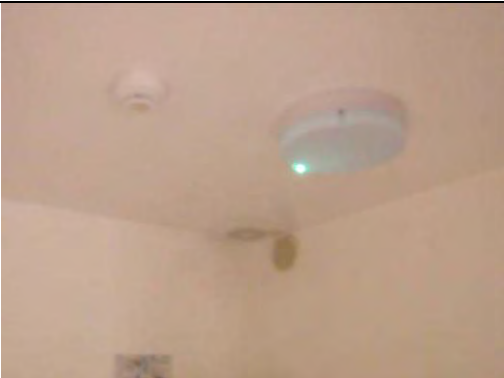
Painted plasterboard ceiling
