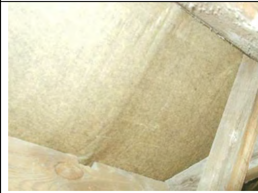
General view above with MMMF insulation above
