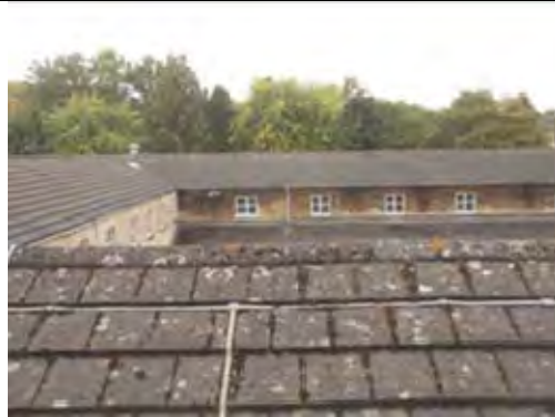
General view of Roof with concrete tiles to roof
