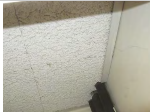
Older style non ACM ceiling
