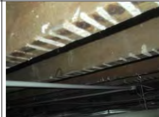
General view above suspended ceiling tiles
