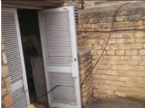
General view of Boiler Room Entrance
