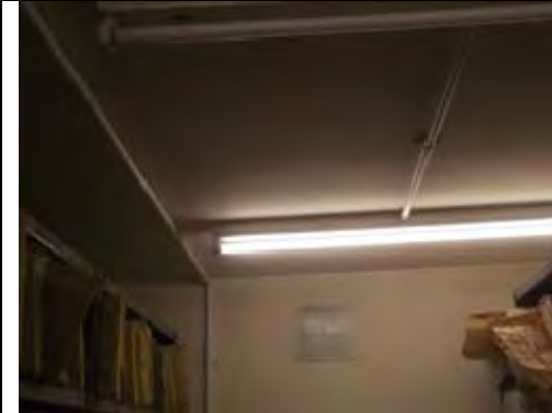
Painted plastered walls and ceiling
