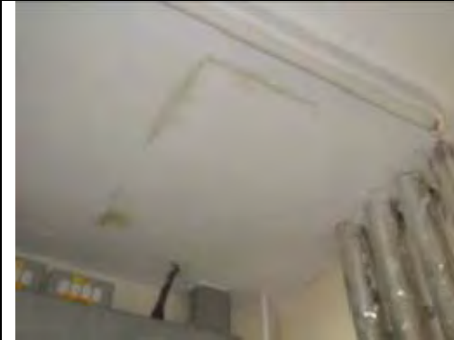
Painted plastered ceiling and non ACM lagged pipes
