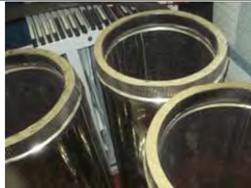
Modern non ACM twin walled flues
