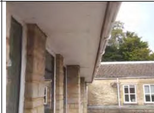
Insulation board soffits CDCOTR/9 NADIS
