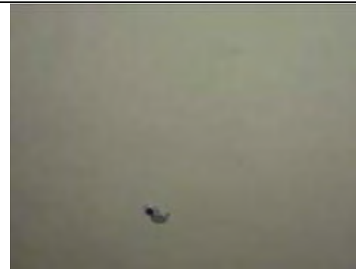
Painted plasterboard ceiling
