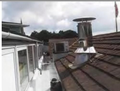
General view of roof
