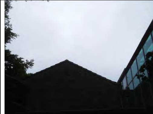
General view of Roof
