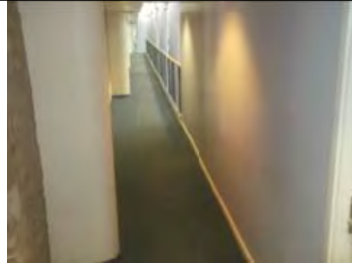
General view of Corridor
