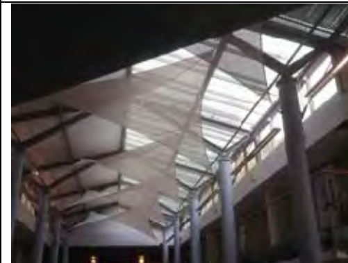
Glass to roof
