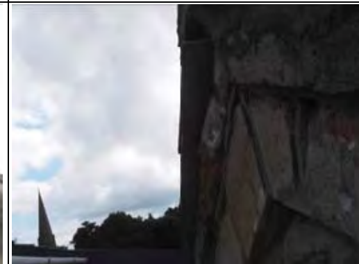
Cement under cloaking to roof CDCOTR/1 Chrysotile
