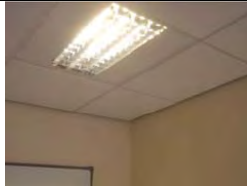
Modern non ACM suspended ceiling tiles
