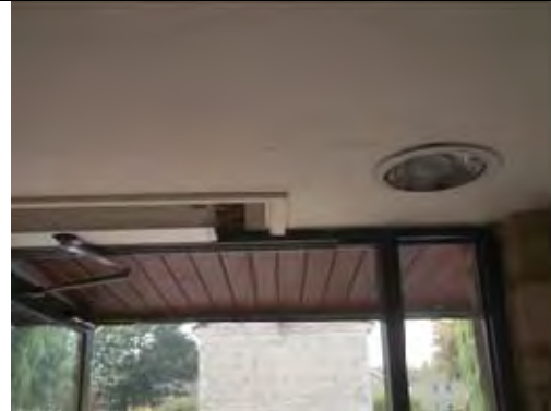
Painted plasterboard ceiling and timber ceiling
