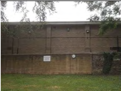
General view of Rear Elevation
