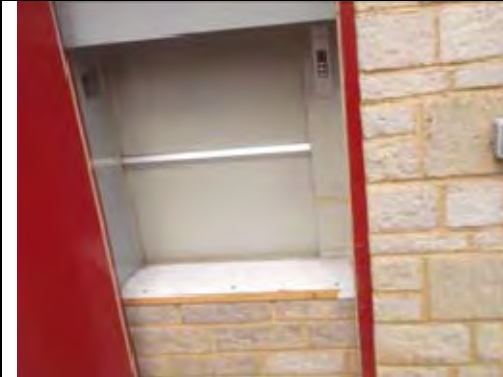
Goods Lift to First Floor 1.67
