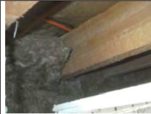
General view above suspended ceiling. MMMF insulation. Non ACM
