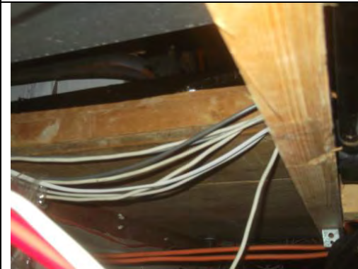
General view above suspended ceiling
