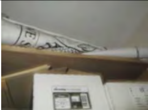
Painted plasterboard ceiling
