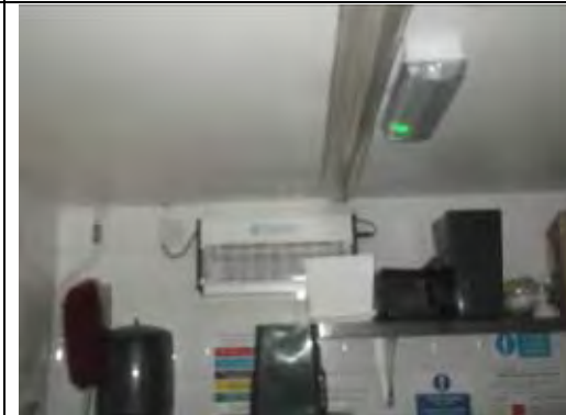
Painted plasterboard ceiling
