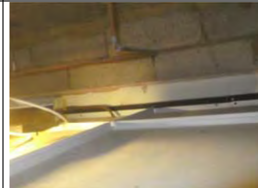
General view above suspended ceiling
