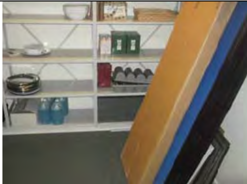
General view of Store 2. Painted plasterboard walls and carpet on concrete floor
