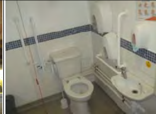
General view of Disabled WC
