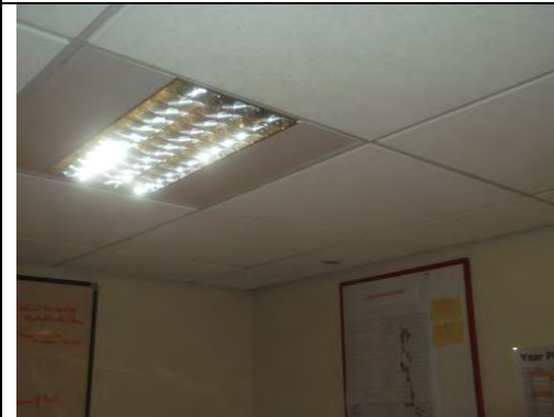
Modern non ACM suspended ceiling tiles with painted plastered walls
