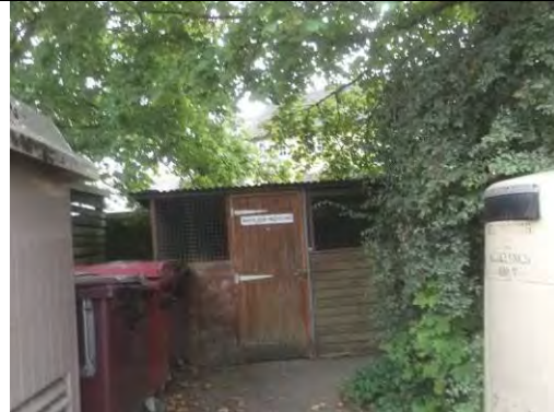
General view of Store
