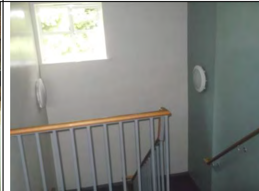
General view of Stairwell
