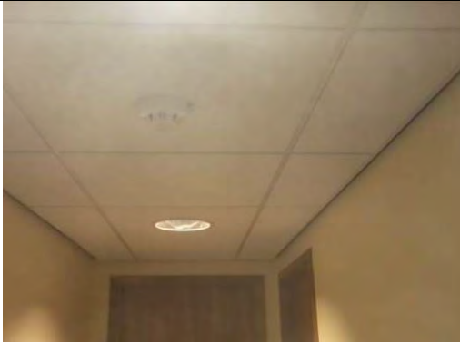
Painted plastered walls and modern non ACM suspended ceiling tiles
