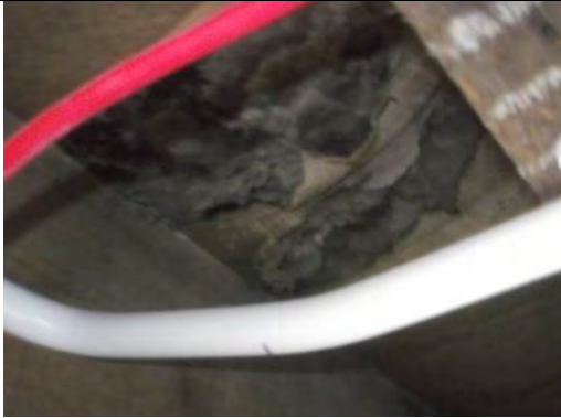
MMMF insulation. Non ACM
