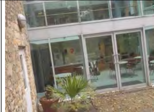
General external view of 0.51 Cafe
