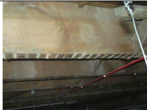
View above suspended ceiling with timber beams
