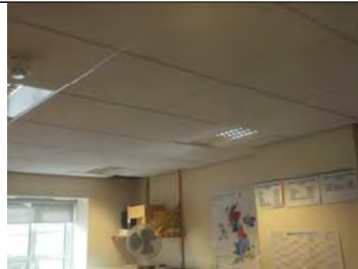
Modern non ACM suspended ceiling tiles and painted plastered and plasterboard walls
