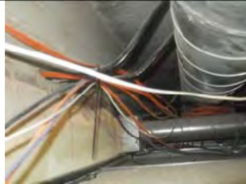
General view above suspended ceiling
