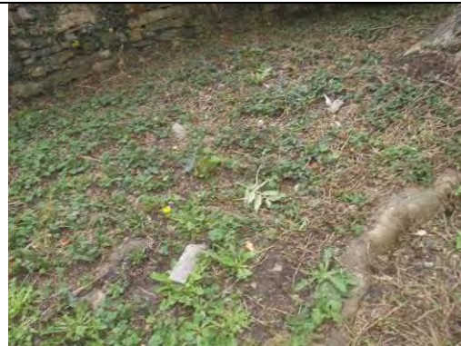
Asbestos cement debris within Garden Removed
