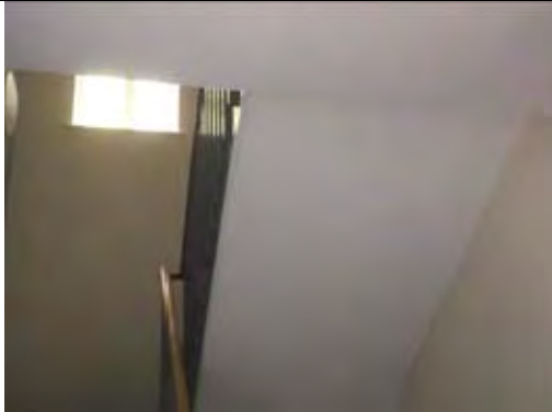
Painted plastered concrete to underside of stairs
