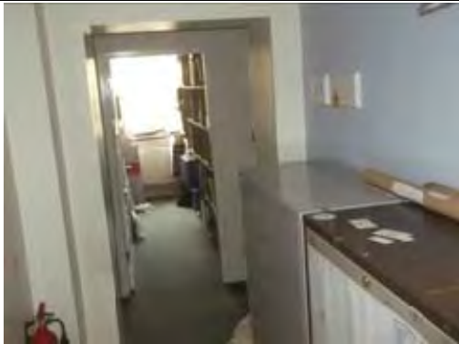
General view of Corridor
