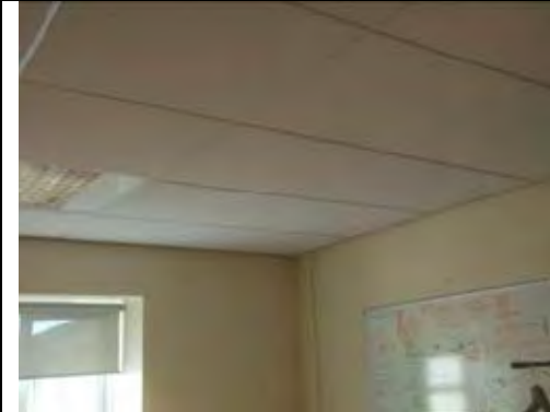
Modern non ACM suspended ceiling tiles
