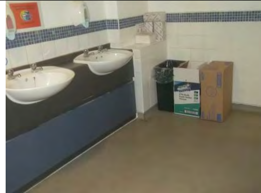
General view of Ladies WC
