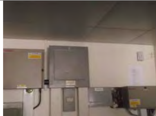
Modern non ACM suspended ceiling tiles and modern non ACM electrics
