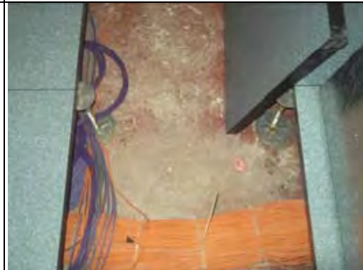
Concrete floor below suspended timber floor
