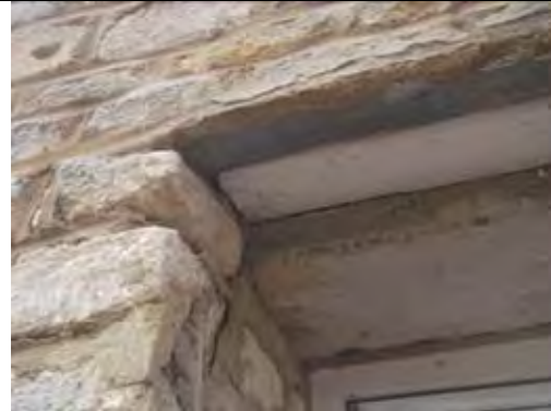
Concrete lintel and timber header to doorway
