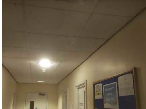
General view of Corridor
