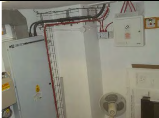
General view of Store 1
