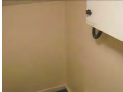
Painted plastered walls
