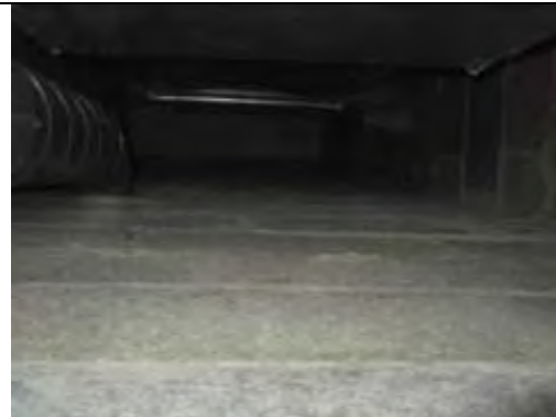
Modern non ACM plant
