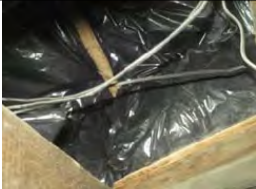
Modern non ACM MMF insulation wrapped in plastic
