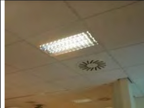
Modern non ACM suspended ceiling tiles
