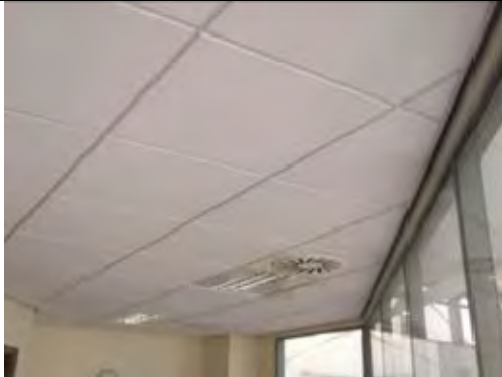
Modern non ACM suspended ceiling tiles
