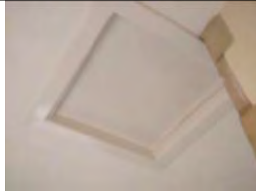
Painted plasterboard ceiling and timber loft hatch
