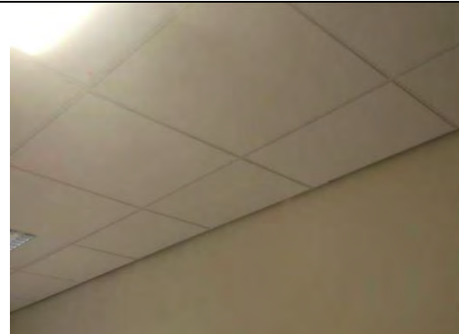
Modern non ACM suspended ceiling tiles and painted plastered wall
