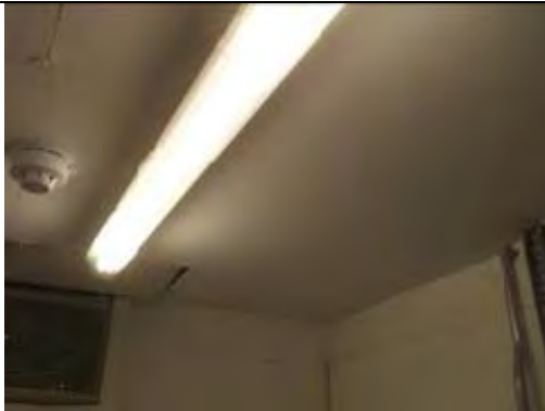
Painted plasterboard ceiling
