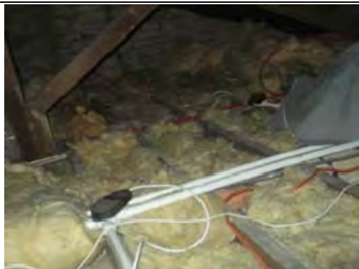
General view within Loft Space with MMMF insulation
