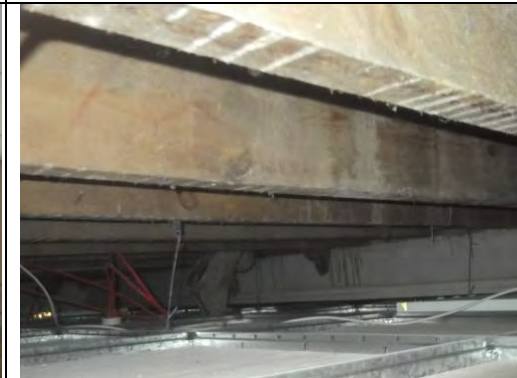
General view above suspended ceiling tiles
