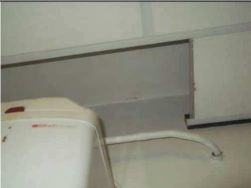
Modern non ACM ceiling tiles
