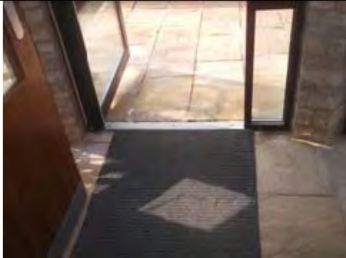
General view of Entrance Hall
