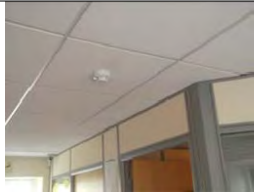
Modern non ACM suspended ceiling tiles
