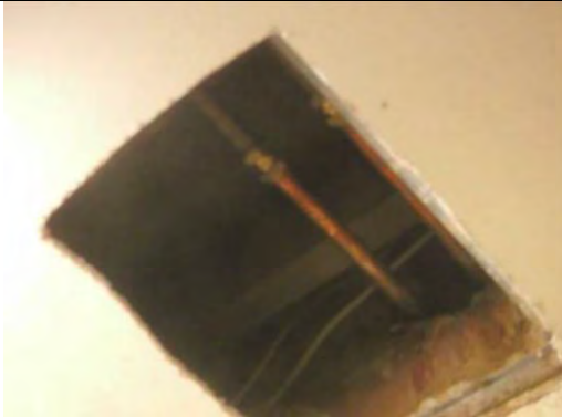
General view above ceiling
