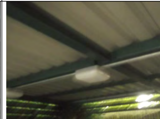
Profiled metal sheet roof
