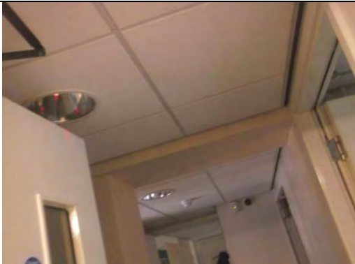
Modern non ACM suspended ceiling
