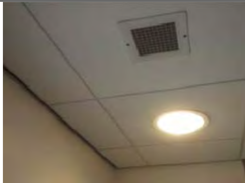
Modern non ACM suspended ceiling tiles
