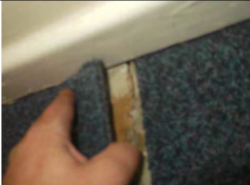
Carpet on concrete
