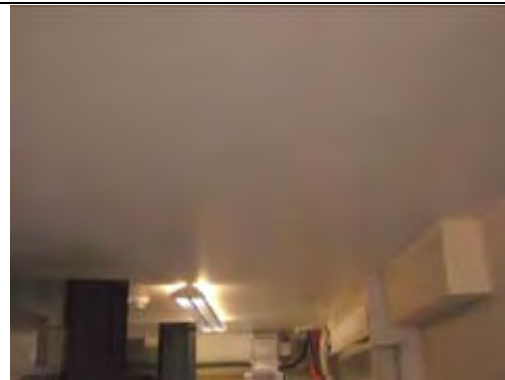
Painted plasterboard ceiling and painted plastered walls
