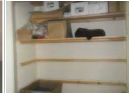
Painted plastered walls
