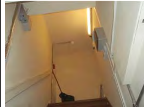
General view of Stairwell
