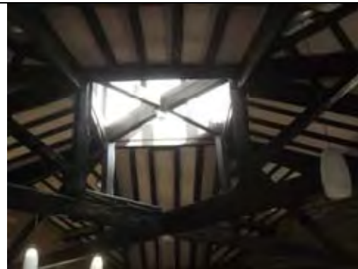
Painted plasterboard lining panels and stone walls
