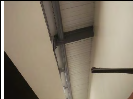
Modern non ACM steel insulated panels to roof
