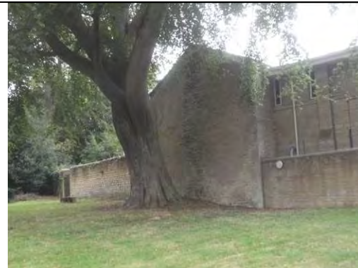
General view of Rear Elevation
