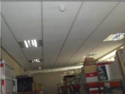
Modern non ACM suspended ceiling tiles
