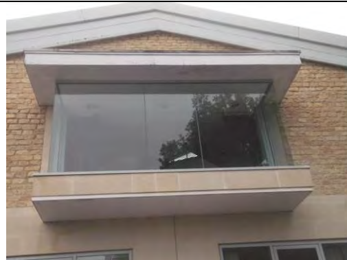
Modern non ACM construction to extension
