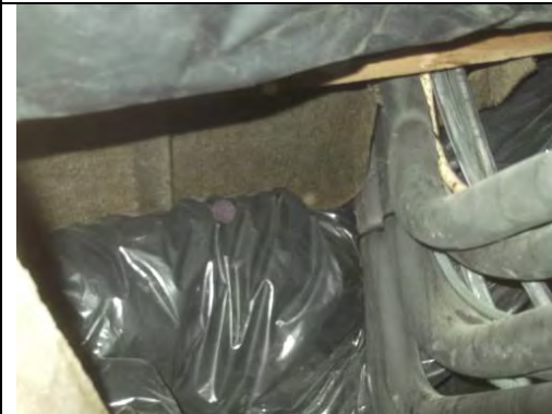
Modern non ACM insulation and modern non ACM roofing felt
