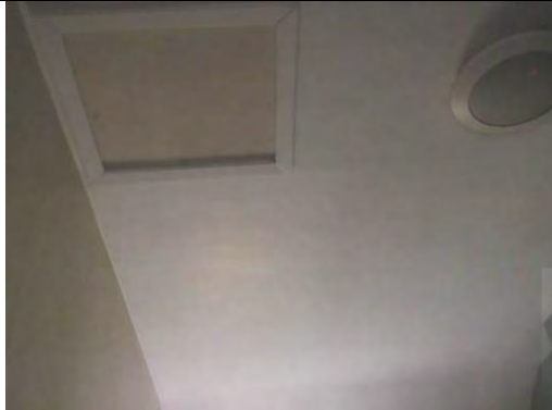
Painted plasterboard ceiling
