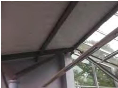
Insulated metal panels to roof
