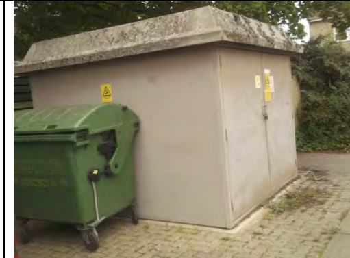
General view of non ACM GRP Sub Station Building
