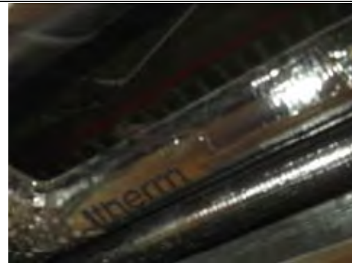
MMMF insulation to pipes with foil wrap
