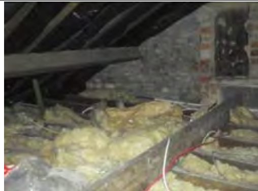
General view of Loft Space
