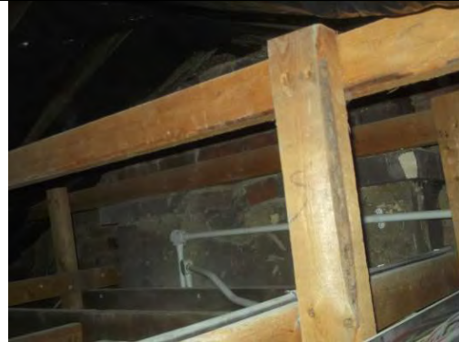
General view above suspended ceiling tiles
