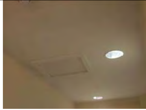
Painted plasterboard walls and ceiling
