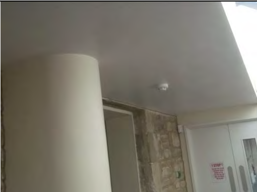
Painted plasterboard ceiling
