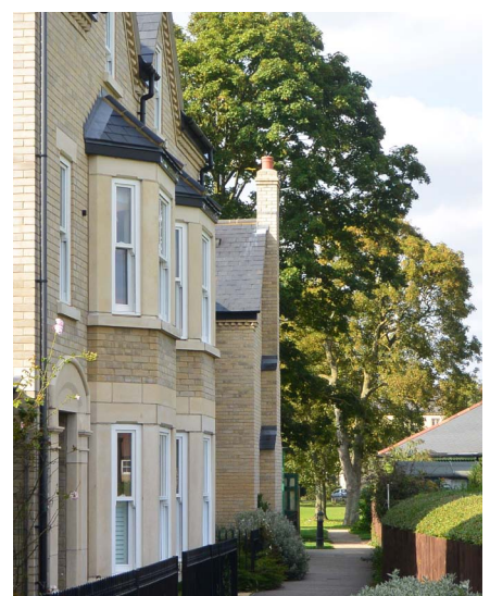
Implemented schemes should clearly distinguish between the public realm and private space
