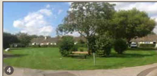
4 Space in front of Sheltered Housing bungalows off Gassons Road
