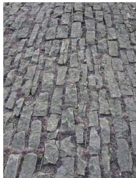
Figure 3.1: Limestone setts in Gosditch Street
