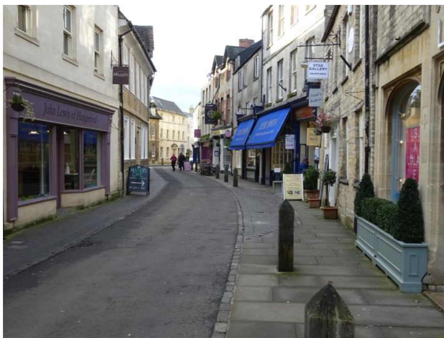
Figure 3.13: Yorkstone flags, granite setts and blue brick paving on Black Jack Street
