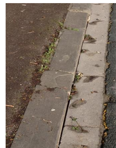
Figure 3.5: Wide top natural stone kerb and channel on Tetbury Road
