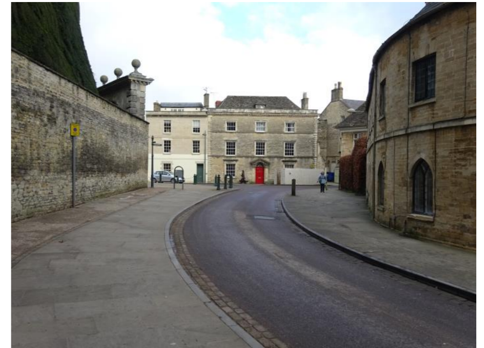
Figure 3.10: Successful natural stone paving scheme in Park Lane using Yorkstone flags and setts and granite kerbs
