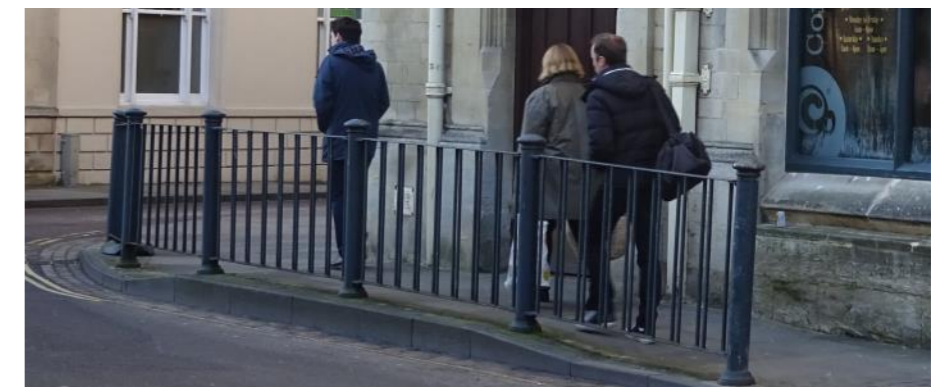
Figure 3.32: Pedestrian Guard Rails at the junction of Castle Street and Silver Street prior to public realm improvement works
