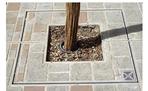
Figure 3.49: Using a recessed metal tray tree grille system allows the paving to extend closer to the trunk of the tree, simplifying the appearance and minimising the potential for trapped litter etc. Image shows 'Adur' tree grille from Green Blue Urban
