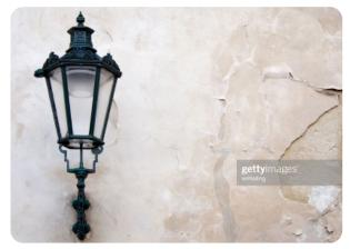
**Unsuitable External Light.** Light is directed sideways meaning that it is spread over a much greater distance. The compact fluorescent bulb is likely to contain wavelengths which are more disturbing to invertebrates than an LED.
