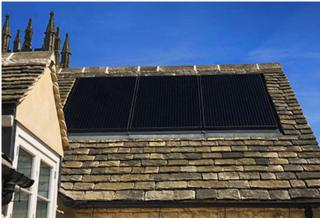
Figure 20: Example image showing the use of solar panels in traditional buildings by making them flush with the tiles.
