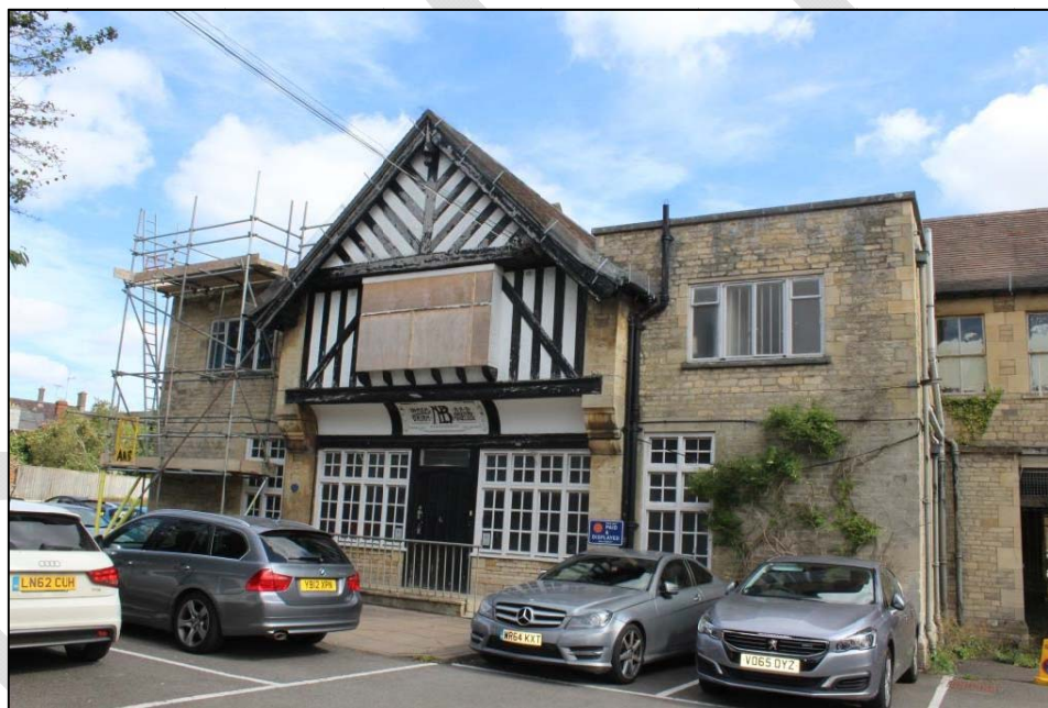
Photograph 1: View of Old Memorial Hospital, view to the north-east
