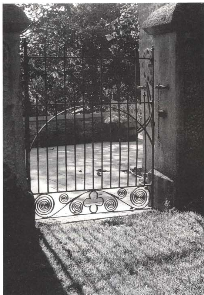
A gate at the Old Forge. The incredibly tight and exuberant scrolls are testimony to the blacksmith's skill, as are the stone gate piers to the mason. Some nice examples of more simple hand forged garden gates survive at Ballinger's Row.
