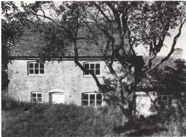
This cottage in Bleakmoor is a good and quite typical example of those found in the village. The building is constructed entirely of local materials but its simple fenestration is enhanced by cambered stone door and window heads.
