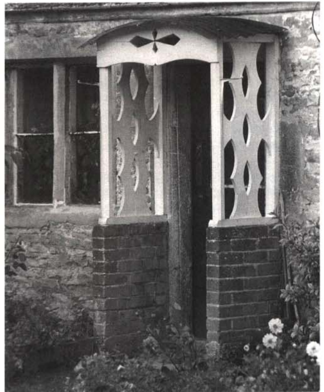
Church Row. The unusual porches with their shallow corrugated iron roofs and pierced side panels are primitive but very pleasing.
