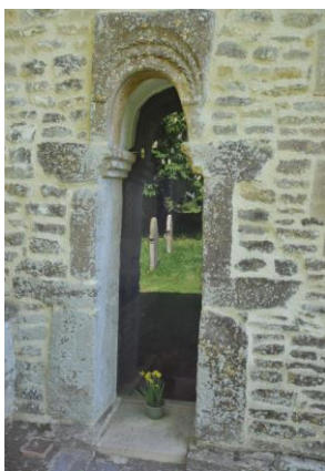
Figure 9: The Saxon doorway, All Saints Church
