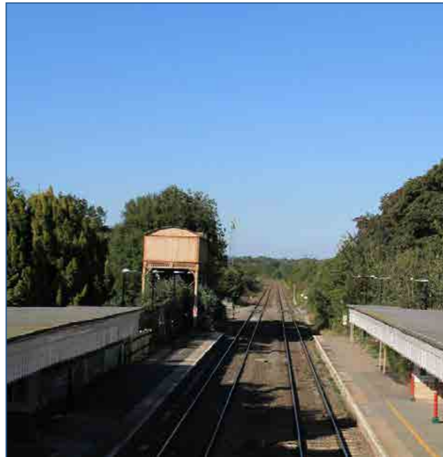
Kemble Station and water tower. Photo Credit: Anne Wilton
