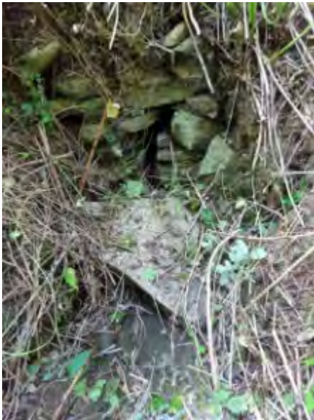
Photograph 12 – The headwall of the pipe joining Drain E after clearing
