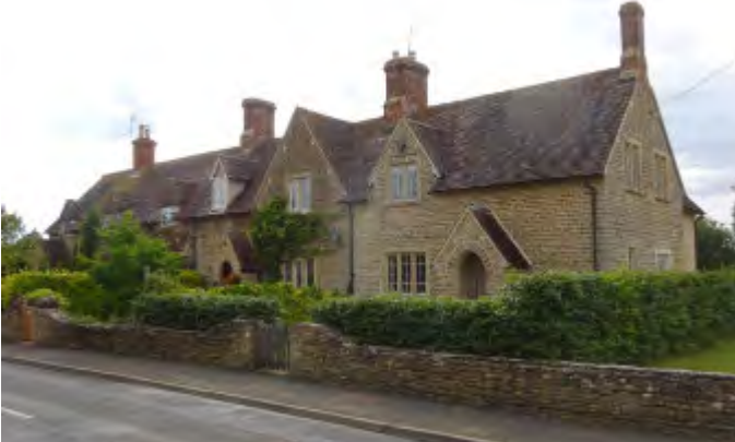
Figure 8.4 Existing row of terraced houses
