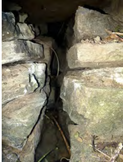
Photograph 15 - Inside the dry-stone outfall from Pipe B
