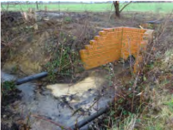
Photograph 8 - Headwall from Pipe C into Drain C (January 2024)
