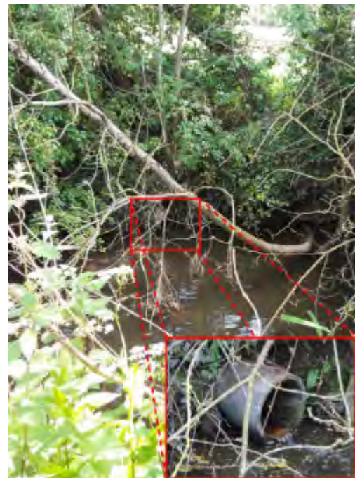
Photograph 13 - Highway drain outfall into Poulton Brook
