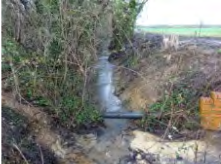
Photograph 7 - Drain C looking North (January 2024)
