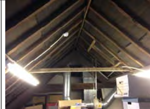
Non ACM lining to roof
