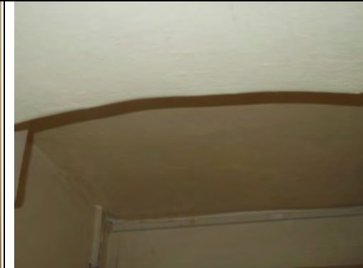
Painted plastered ceiling
