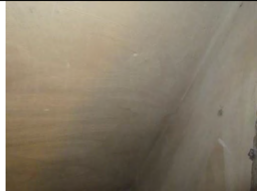
Plastered ceiling and walls
