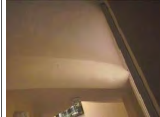
Painted plastered walls
