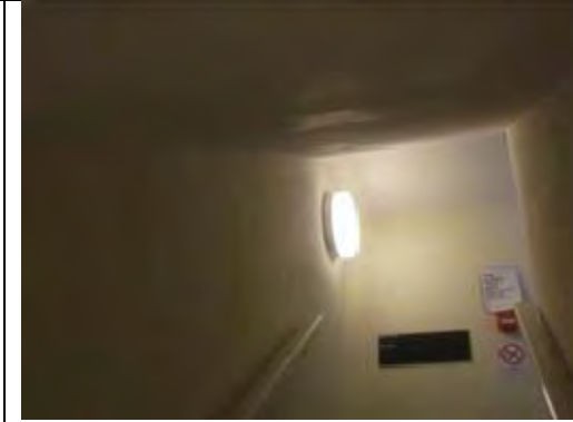
Painted plastered walls and ceiling
