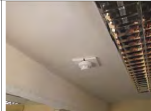
Painted plastered walls and painted plasterboard ceiling
