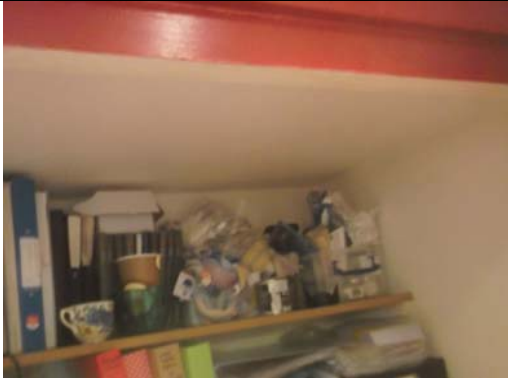
General internal view of Cupboard. Painted plasterboard ceiling
