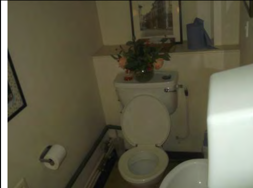
General view of WC. Modern non ACM toilet suite
