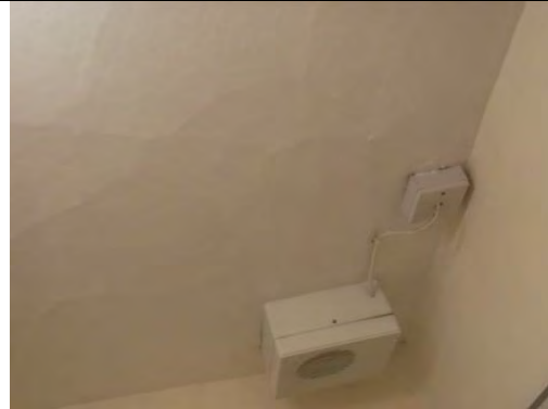
Painted plastered ceiling
