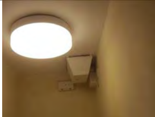
Painted plastered walls and painted plasterboard ceiling
