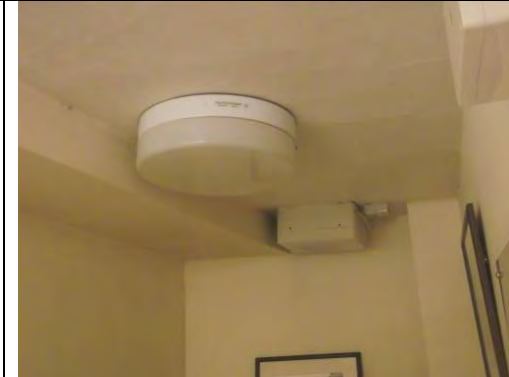
Painted plastered ceiling
