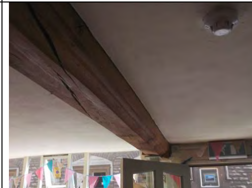
Painted plastered ceiling
