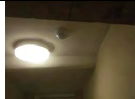
Painted plastered wall and ceiling
