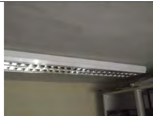
Painted plastered walls and ceiling
