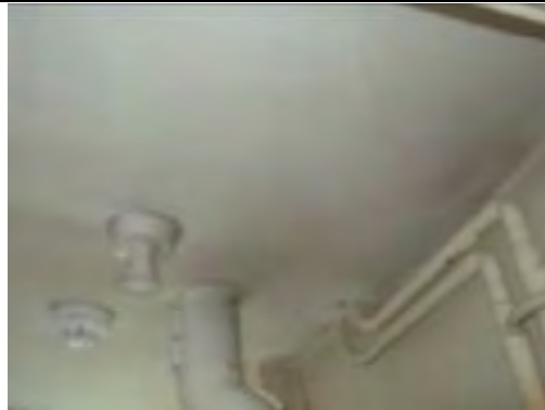
Painted plastered ceiling
