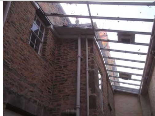
Stone walls and glass roof lights
