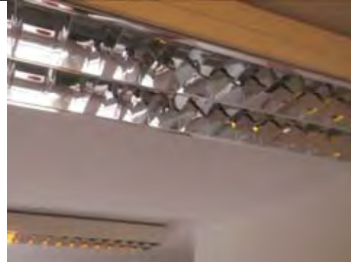
Painted plasterboard ceiling
