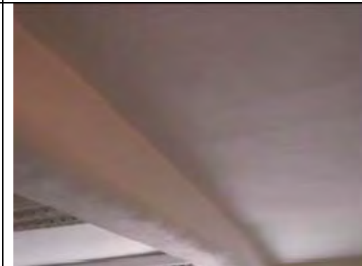
Painted plastered ceiling
