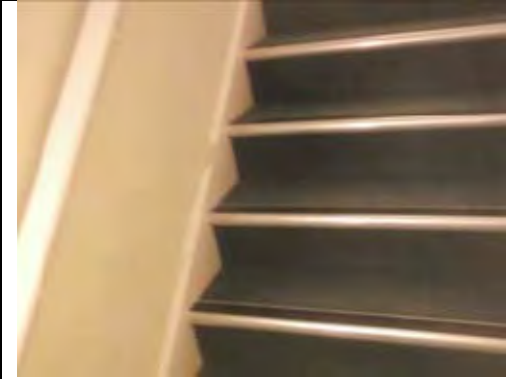
General view of Stairwell. Non ACM stair nosings
