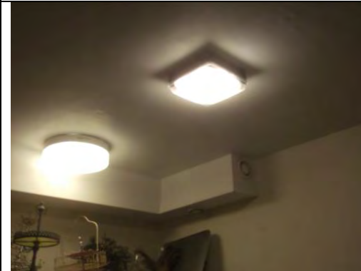
Painted plastered ceiling and non ACM boxwork
