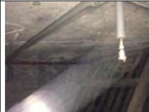
General view of Loft Space and non ACM roof
