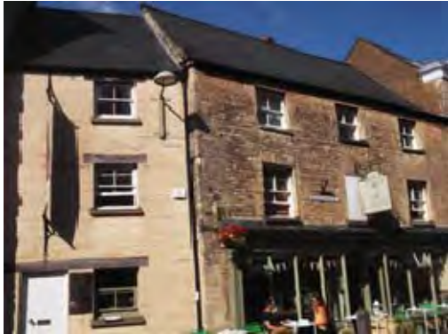
General external view of Black Jacks
