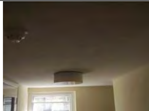
Painted plastered ceiling
