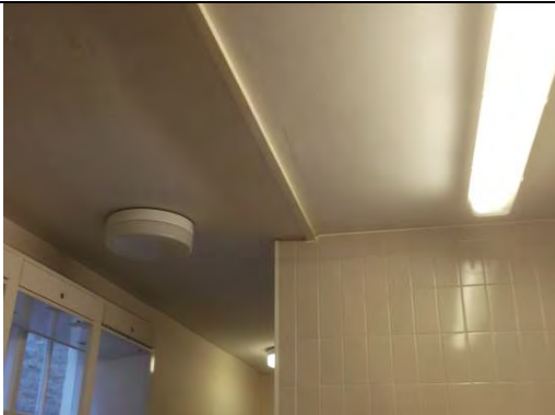
Painted plasterboard ceiling
