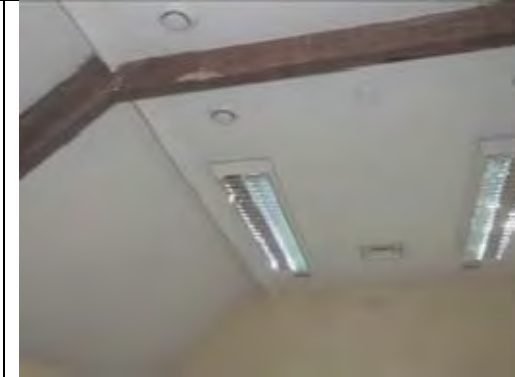
Painted plasterboard ceiling
