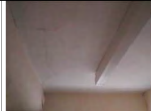
Painted plastered walls and painted plasterboard ceiling
