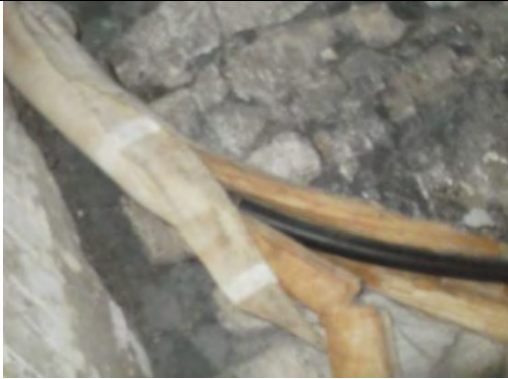
MMMF insulation. Non ACM
