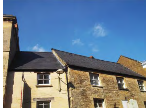
Stone walls and non ACM roof tiles
