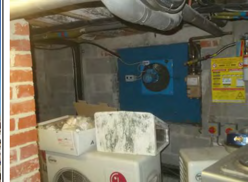
General view of Basement
