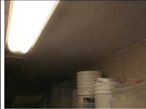
Painted plastered ceiling
