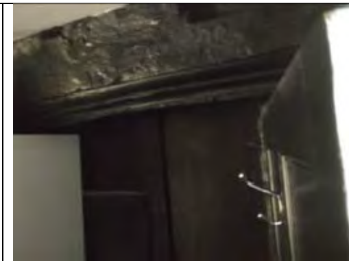
Timber paneling to cupboard beneath stairs
