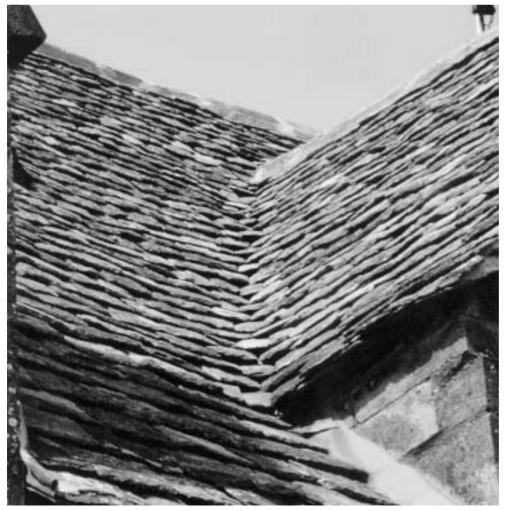
A fine swept valley on a newly-laid roof in Chipping Campden. This detail requires the most skilled craftsmanship in its construction, involving the careful shaping and fixing of the wedge shaped slates in the valley. Often, modern roofers omit this and insert a closemitred or open lead valley. Although both of these are cheaper to construct, neither appear as satisfactory as the traditional valley and are best avoided.
