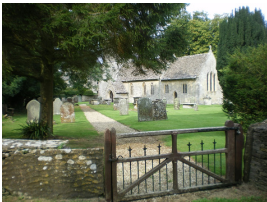
Figure 6: The Church of All Saints is Grade II* Listed and has Norman foundations, with fourteenth century alterations and nineteenth century restoration works. There are numerous listed chest tombs and other monuments within the churchyard.
