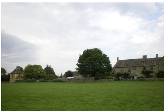
Figure 7: The Manor House is Grade II Listed and dates to at least the sixteenth century, but it is largely seventeenth century. It is typical of a higher status Cotswold vernacular house of that period, with stone tiled roof, large gables, stone cross-mullioned windows and Tudor-arched doorways. To the west there are further listed farm buildings relating to the Manor.
