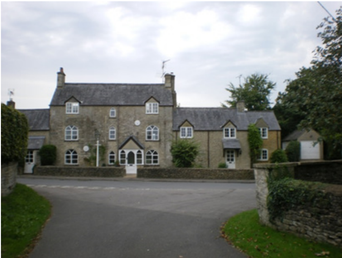
Figure 17: An unlisted cottage, with a blue slate roof, and distinctive arch-headed windows.
