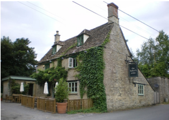
Figure 14: The Bakers Arms pub (Grade II Listed) dates to the eighteenth century.
