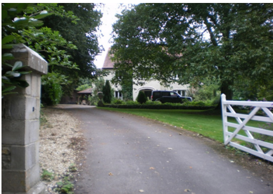
Figure 12: The Old Vicarage dates to the 1920s, and was designed by the notable local architect V A Lawson. It, unusually for the village, is roughcast rendered.
