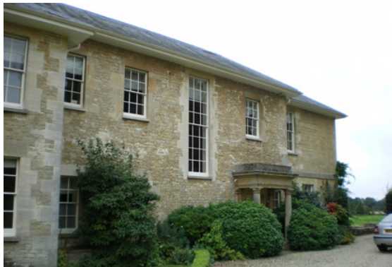
Figure 9: Somerford Keynes House (Grade II Listed) dates to 1804 and is a large house built in the classical style, with overhanging hipped slate roof, sash windows and a Doric porch. The house is set within attractive grounds, open to the former parkland to its west.
