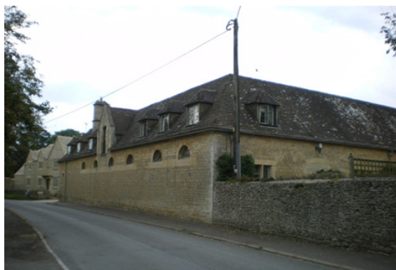
Figure 11: The large stable block (Grade II Listed) adjacent to the Dower House, built in about 1920, has a plain clay tiled roof, with hipped dormers, and high level half-round windows set within stone surrounds.
