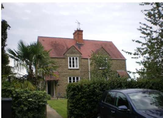
Figure 8: A pair of unlisted late nineteenth century cottages to the north of the Church.
