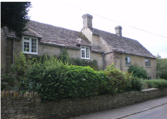
Figure 16: An unlisted cottage, with an attractive stone tile roof.
