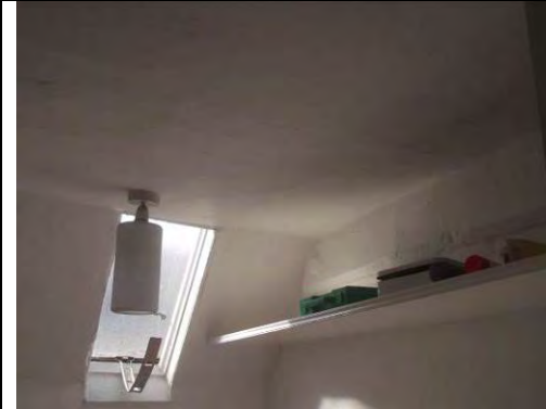
Painted plastered ceiling
