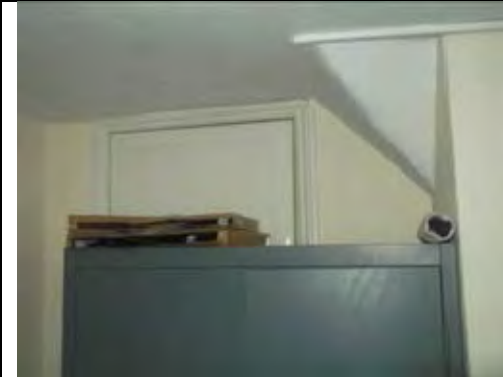
Painted plastered wall and timber door
