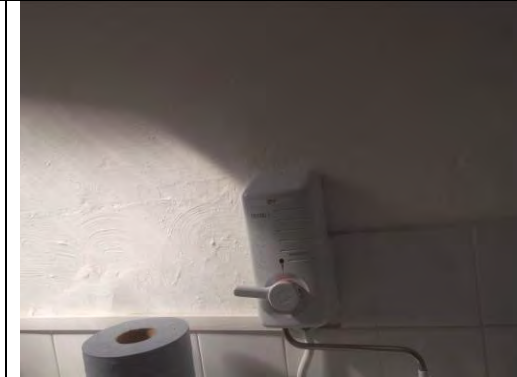
Textured coating to wall AHC/7 NADIS
