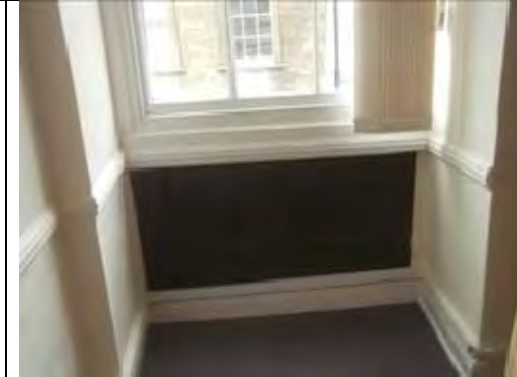
Timber panels to window reveal
