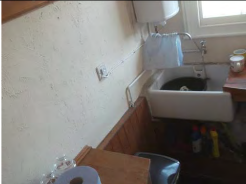
General view of Kitchen. Textured coating to walls AHC/4 NADIS
