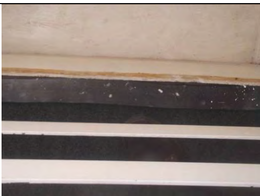
Insulation board to edge of landing floor AHC/1 Amosite/ Chrysotile
