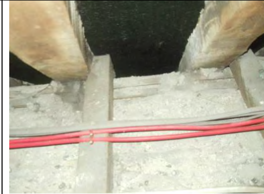
Loft floor with lathe and plaster ceiling below
