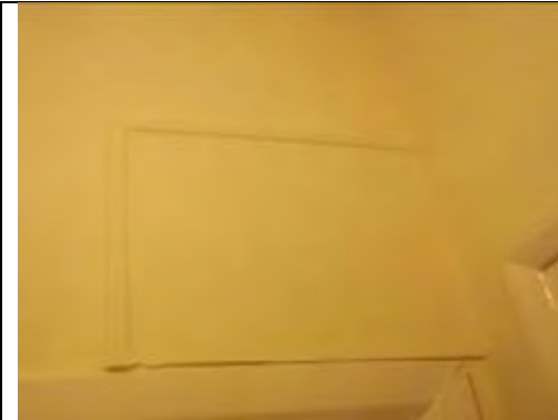
Painted non ACM panel
