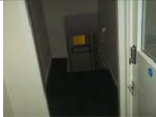
General view of Corridor
