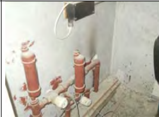
Non ACM heating pipes
