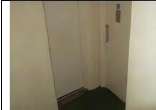
General view of Lobby
