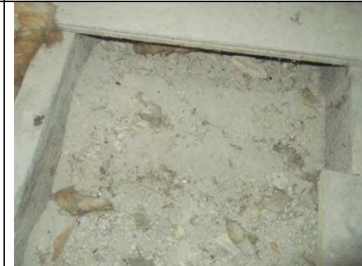
Loft floor and lathe and plaster ceiling below
