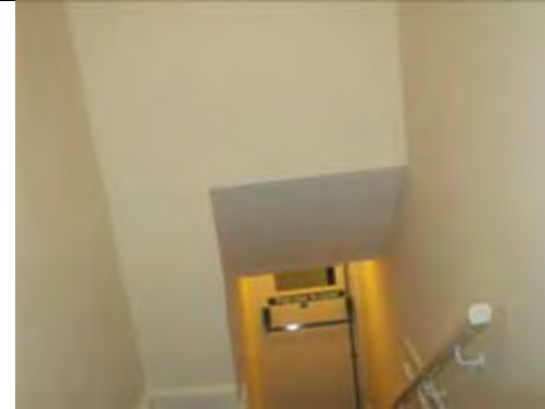
General view of Stairwell
