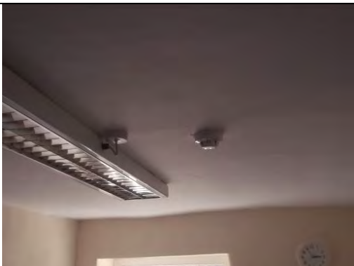
Solid painted plastered walls and painted plastered ceiling
