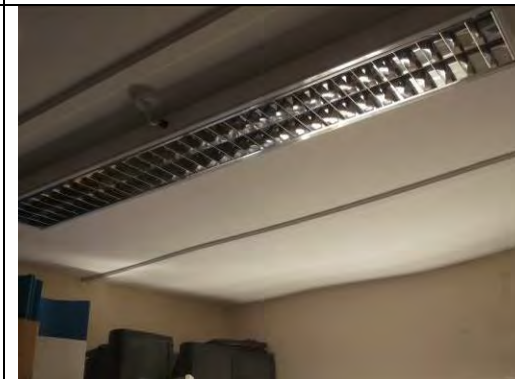
Painted plastered ceiling
