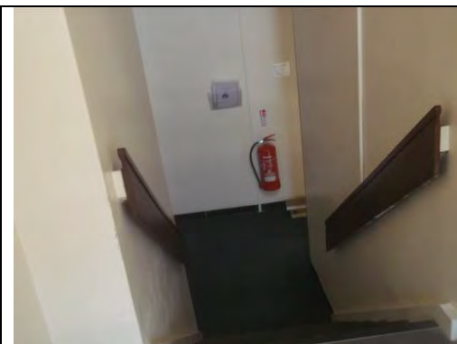
General view of Stairwell
