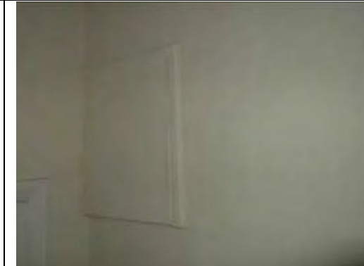
Painted plastered walls and non ACM panel to wall
