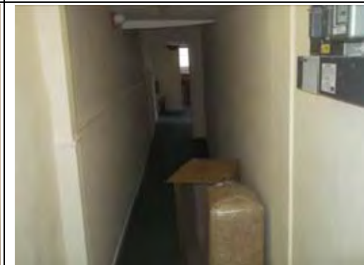
General view of Second Floor. Corridor
