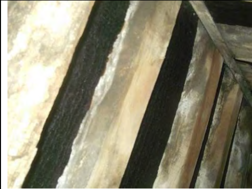
Non ACM roofing felt
