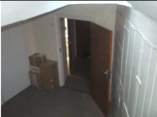
General view of Corridor
