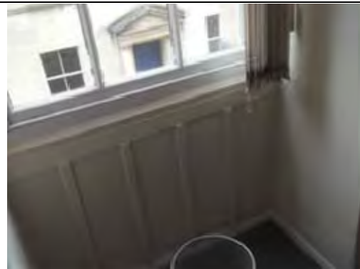
Painted timber panels to window reveal
