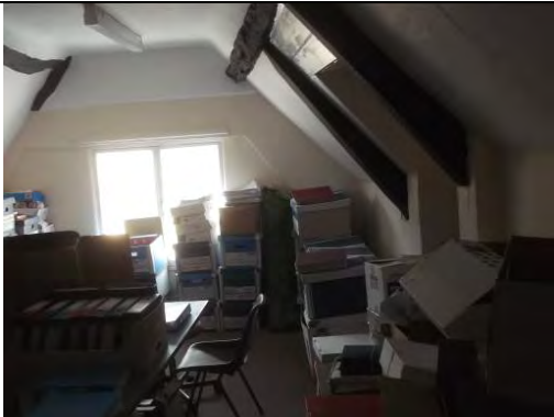
General view of Office 11
