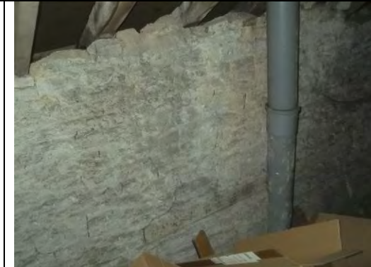
General view within Cupboard
