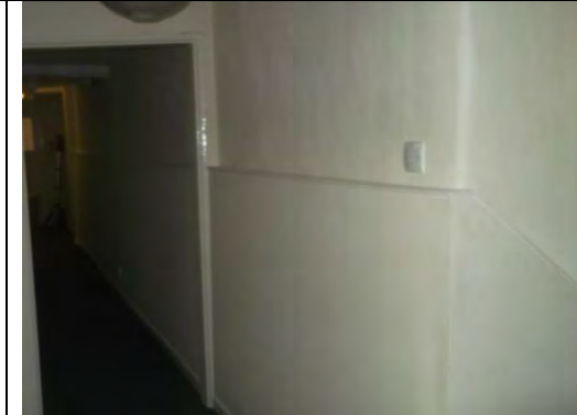
Insulation board to corridor AHC/5 NADIS
