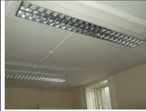
Painted plastered ceiling
