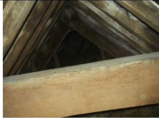
Timber construction to roof
