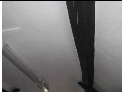
Painted plastered ceiling
