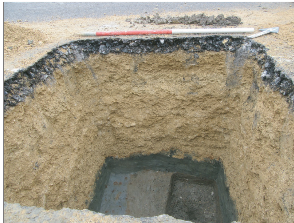
Trench 2, looking north-west (1m scale)
