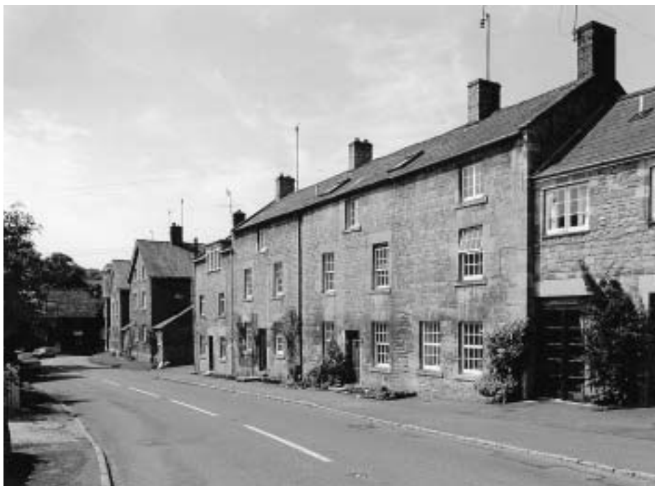
Two sets of nineteenth-century terraces in Lower Street, the near group dating from around 1840, while the others in Lower Terrace date from 1851.
