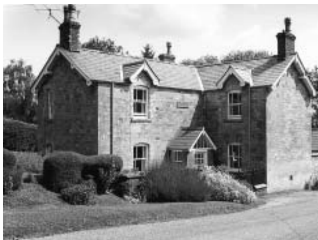
Orchard Cottage in Draycott Lane has a Victorian architectural character resulting from the arched windows with brick surrounds and the decorative bargeboards.
