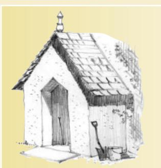
This front porch at Doughton has a stone slate roof crowned by a carved stone finial. The walls are roughcast rendered, which is a typical treatment of walls in the Tetbury area.
