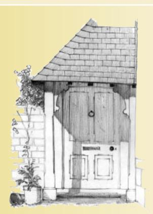
A Victorian porch on the Williamstrip Estate. The robust posts are stop-chamfered and the brackets distinctively shaped.
