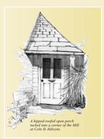
Simpler porches or open loggias are found protecting service entrances. The loggias were usually supported on timber posts set upon tapered stone plinths, and were roofed in corrugated iron as well as Cotswold stone slates, plain clay tiles or blue Welsh slates.
