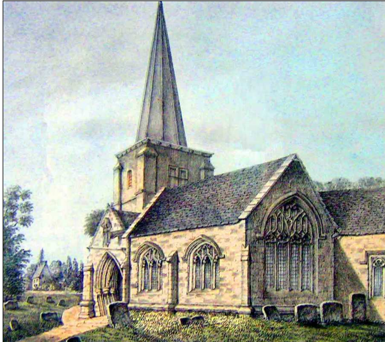
Plate 5.2: Unnamed sketch of All Saints Church dated c1843 showing the distortions of the south porch prior to its reconstruction (Source: http://thames.me.uk/ ).
