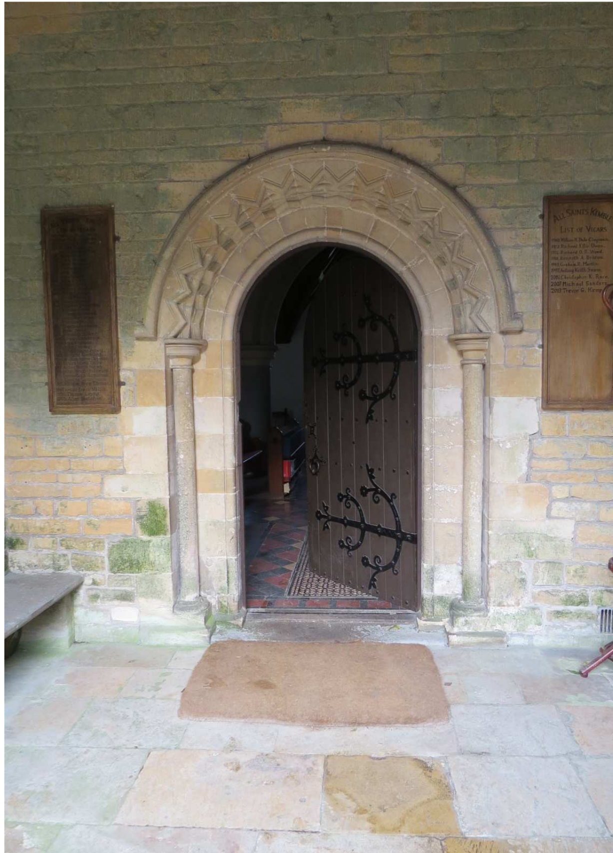
Plate 5.4: The reset arch doorway in the south porch of All Saints Church with distinctive Norman chevron pattern.
