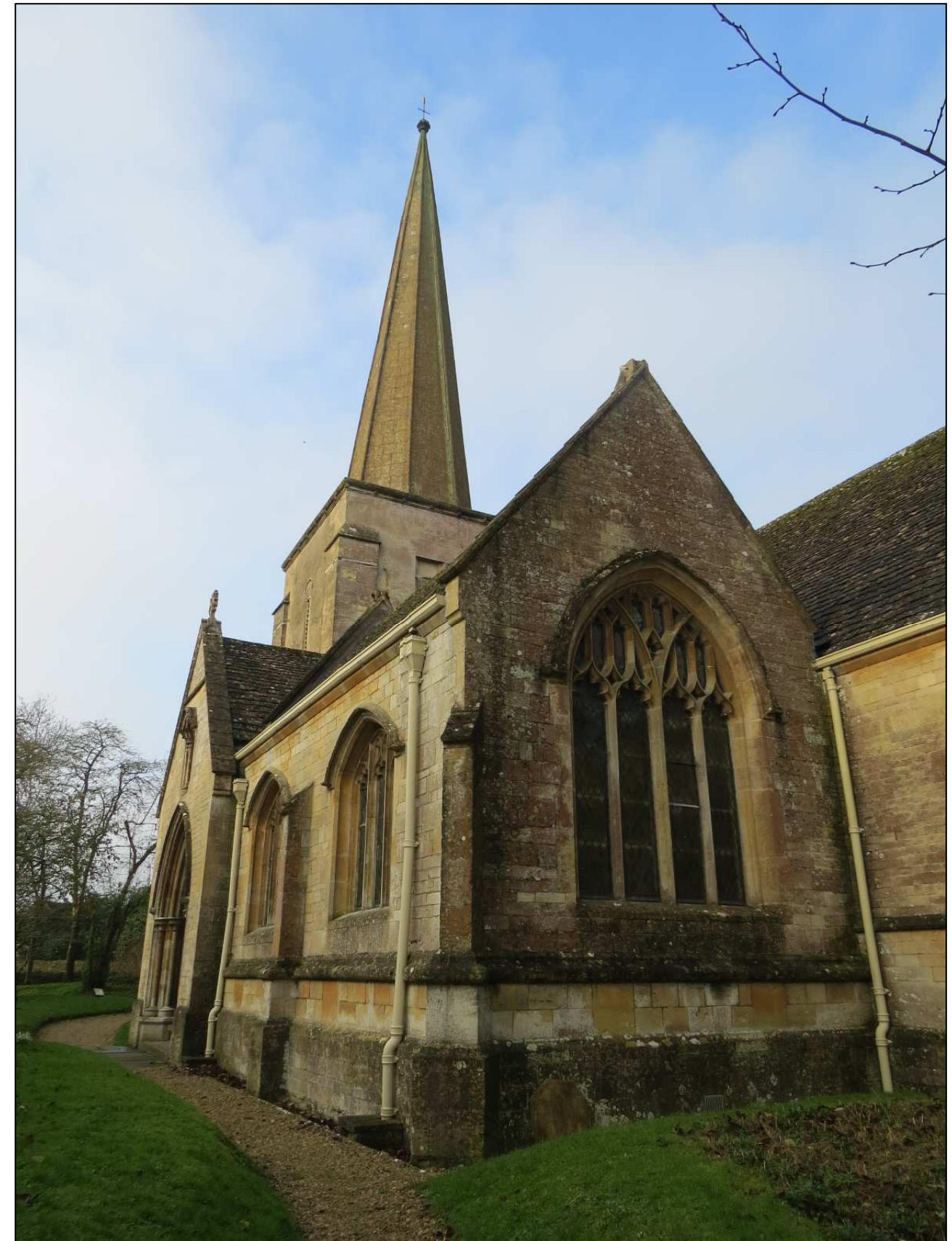
Plate 5.1: All Saints Church with the southern porch and aisle in the foreground.
