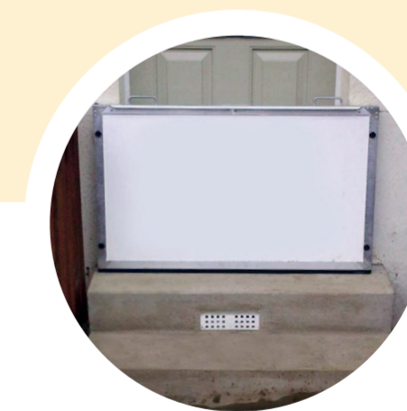
7. At Courtbrook 7 properties have been given flood-protection products. This includes door guards and airbrick covers.
