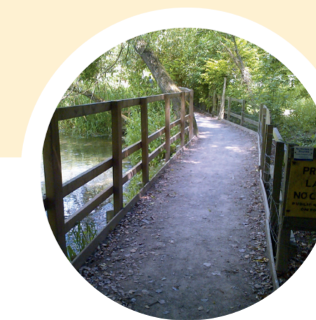
6. Near Dilly's Bridge the public footpath was raised. This reduces the flood risk to Courtbrook.
