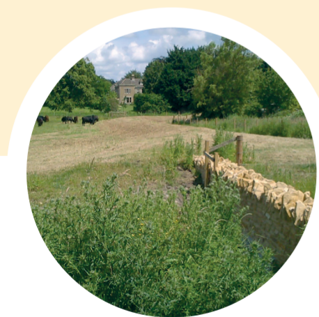
1. In Waterloo Meadow an earth bund was built. This protects Milton Street and cuts off the flow of water onto London street.
